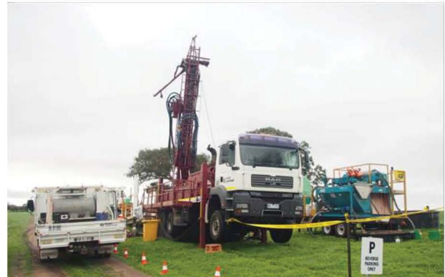
No sumps – closed loop system
