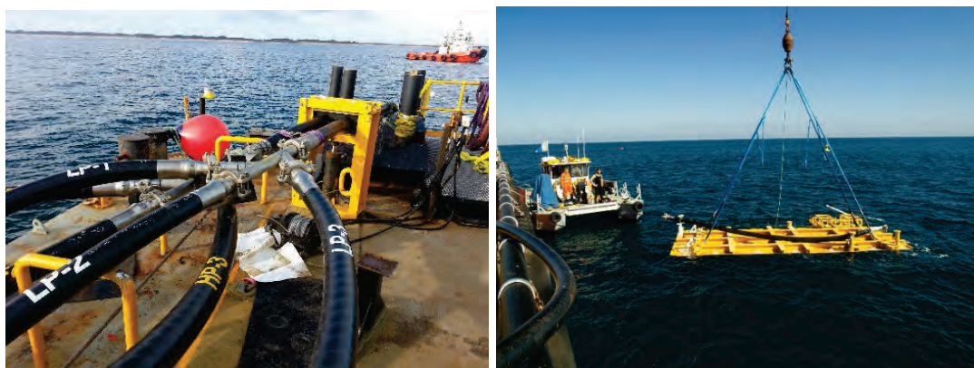
Installation of Interconnection pipes (left) and installation of pod mudmat (right)
