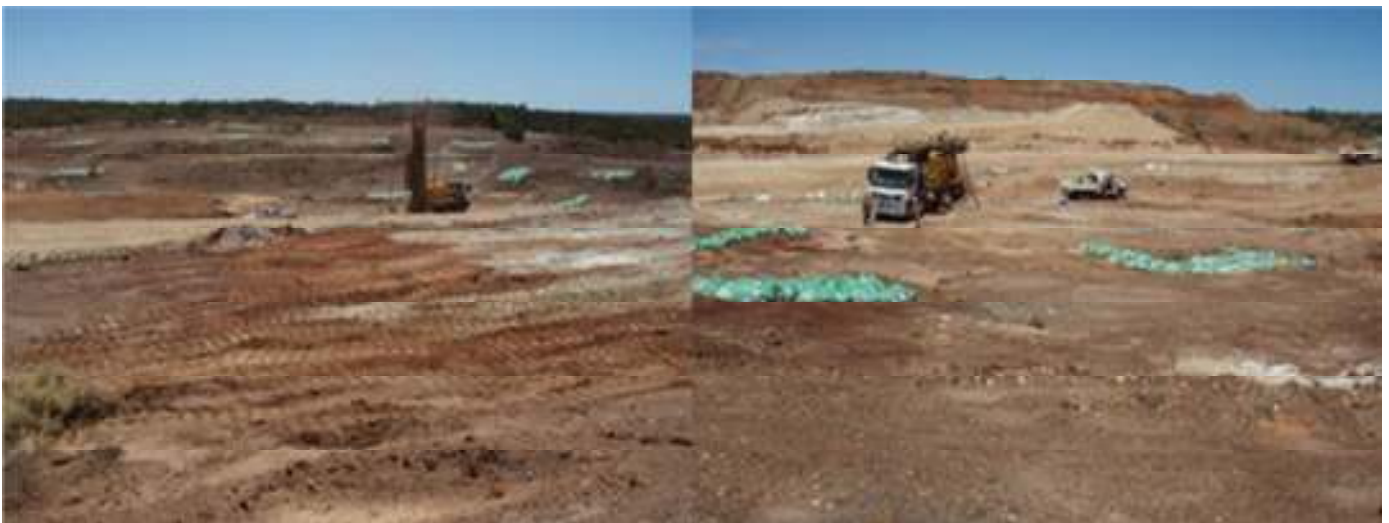
Figure 3 & 4: Gwendolyn Pit 'B' Photo During Grade Control – Looking North-east and South-west
