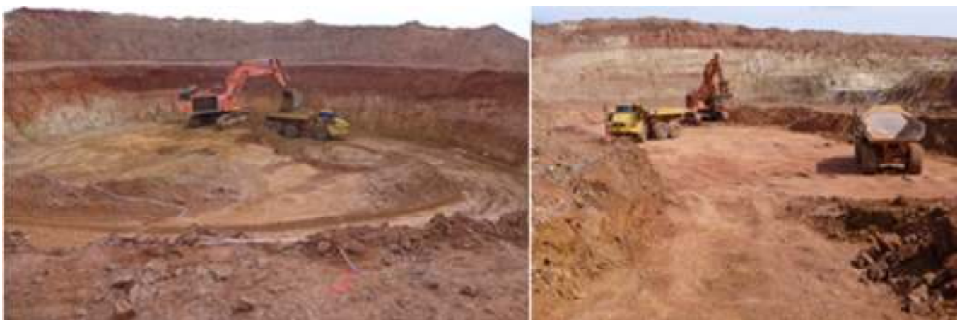
Figure 13 & 14: Gwendolyn Photos of Pits ‘A&B’ Excavations
