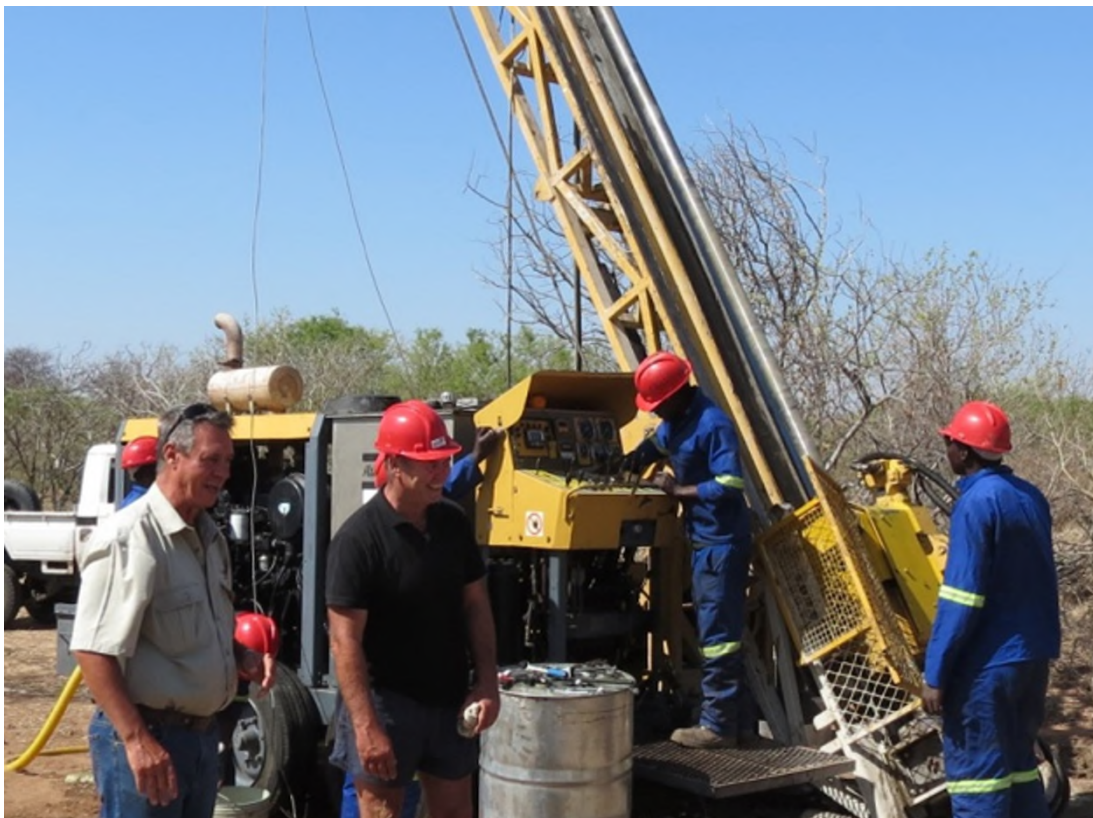
Diamond drilling underway at Mahumo Project
