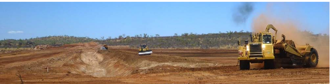
Figure 42: Activity at the TSF. Above two images show keyway construction.
