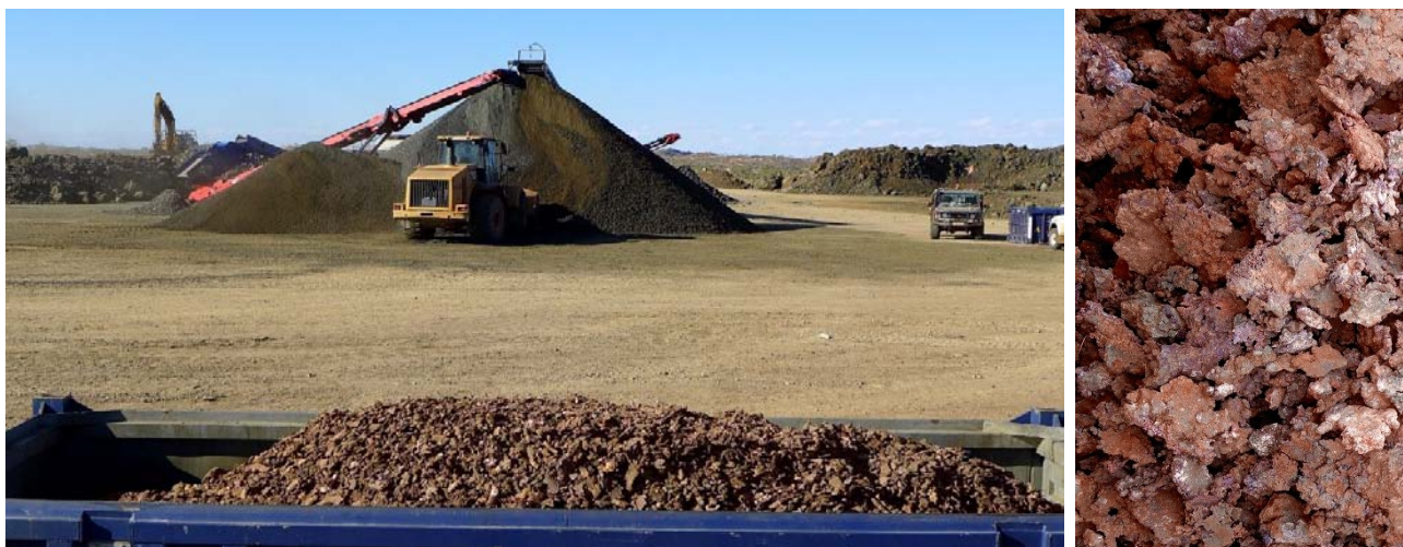
Figure 52: Mobile crusher in operation, with container full of native copper concentrate (foreground) straight from the crusher screens estimated 85-95% Cu and close-up of product (right),
