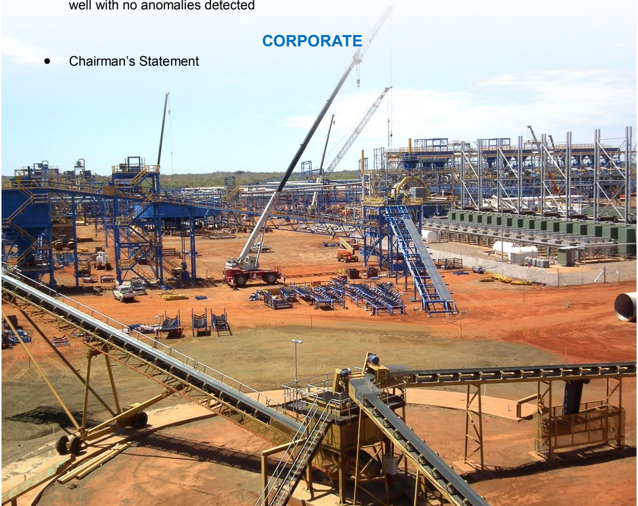
Figure 1: Rocklands Process Plant - major components installed, structural completion underway.
