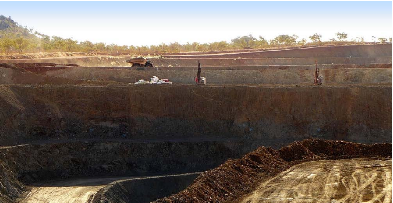
Figure 8: View to north-west showing all three stages of the Las Minerale Pit; Deepest pit is LM1; blast-hole drilling on the shoulder of the LM2 Pit floor and in the background; LM3 Pit (final pit) walls.
