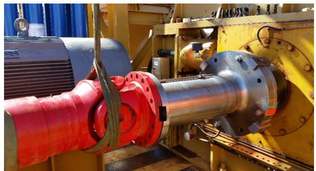
Figure 25: Installing shear couplings
