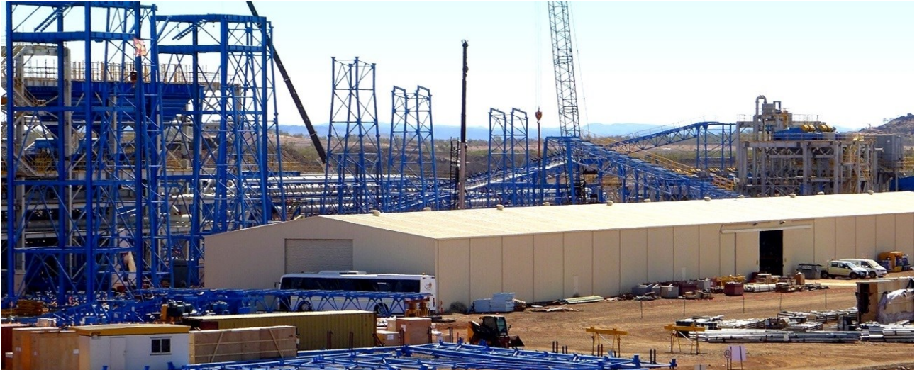
Figure 24: Gravity Jig Building transfer infrastructure and Process Stores Warehouse.
