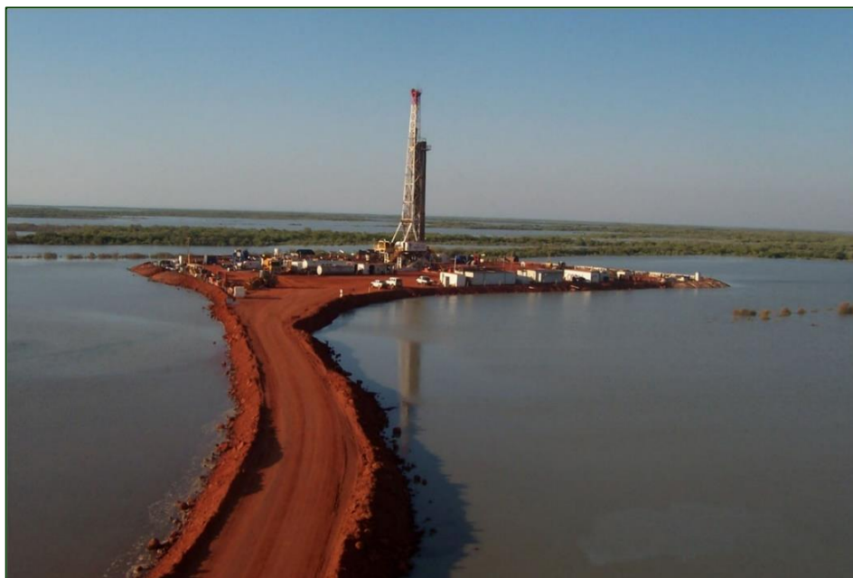
The original causeway at Stokes Bay-1. The remediation of this causeway and at Point Torment-1 will be required before any workover campaign.
