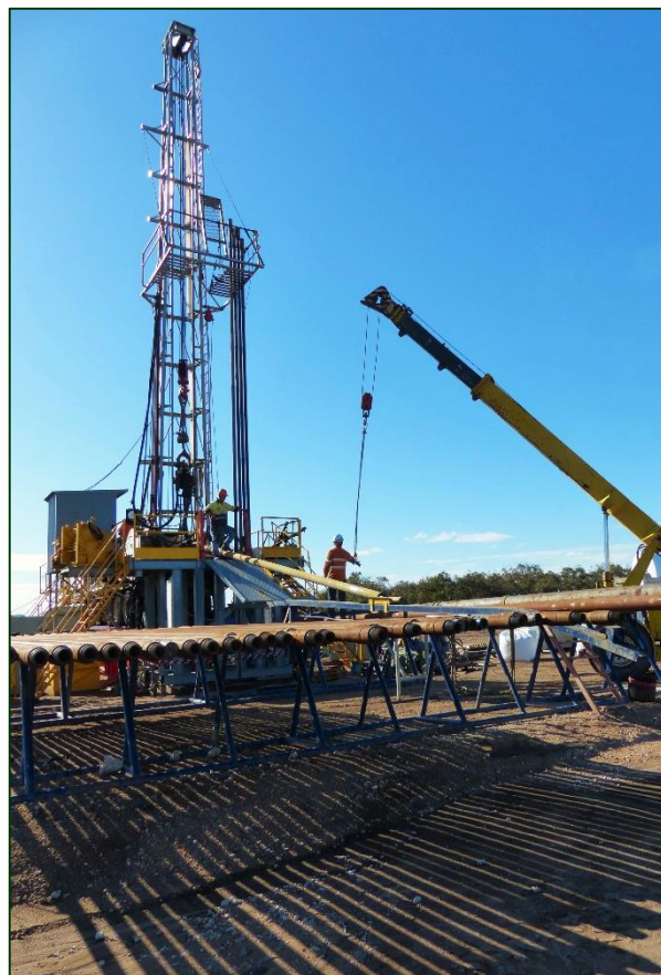
DCA Rig 7 and personnel drilling into the Bookara Sandstone.
