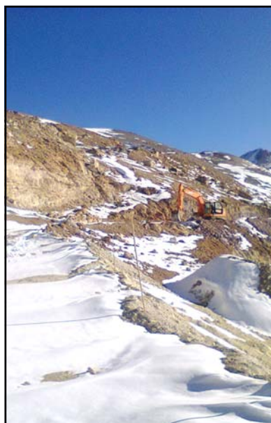
Nueva Esperanza, Chile, access road construction, winter 2014
