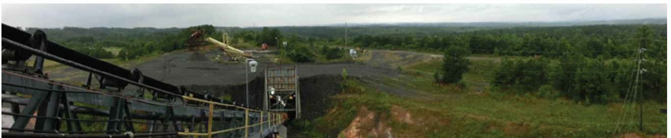
Figure 4. ROM pad at Kodiak Project.
