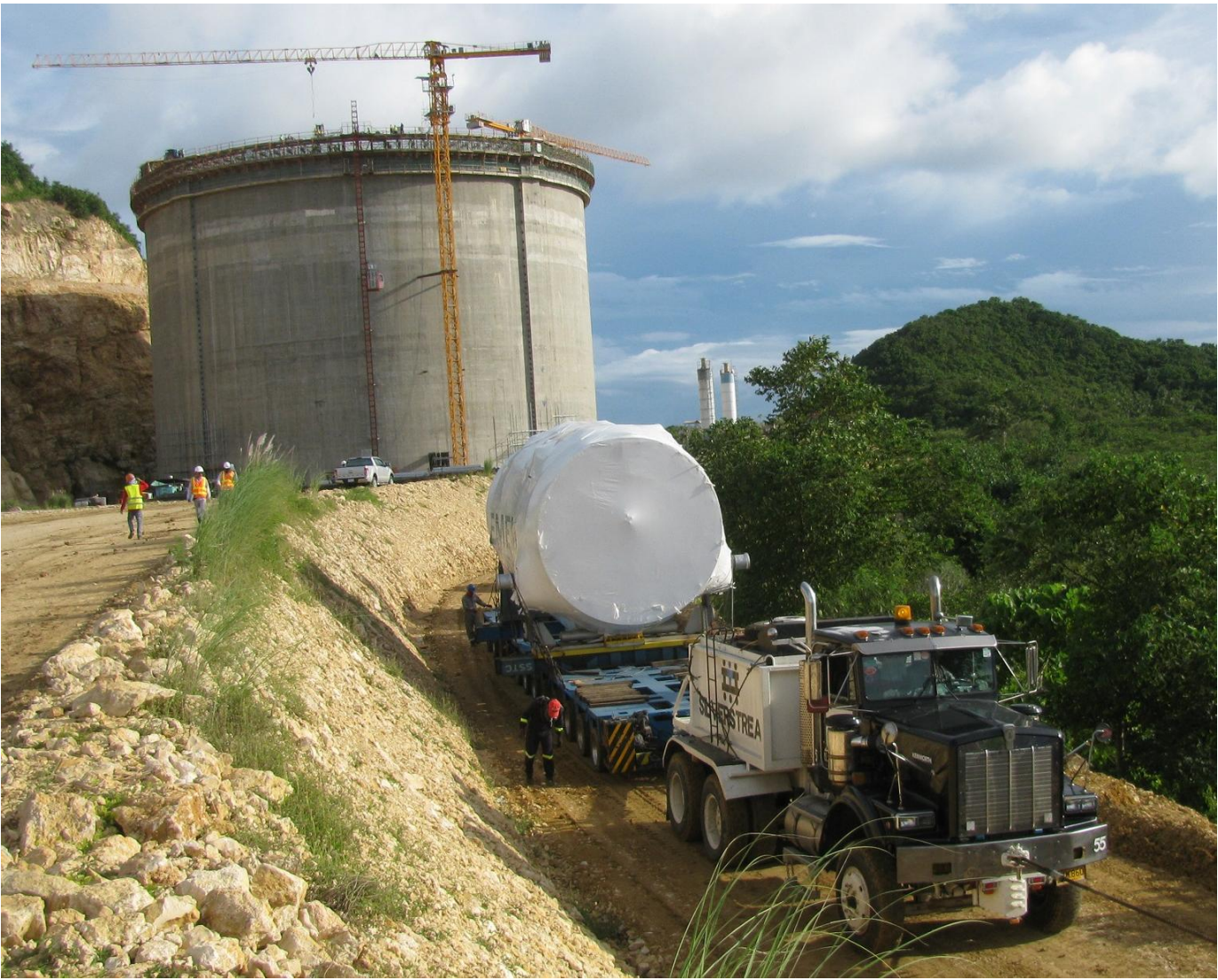
Unloading of Second 200MW Gas Turbine and Generator
