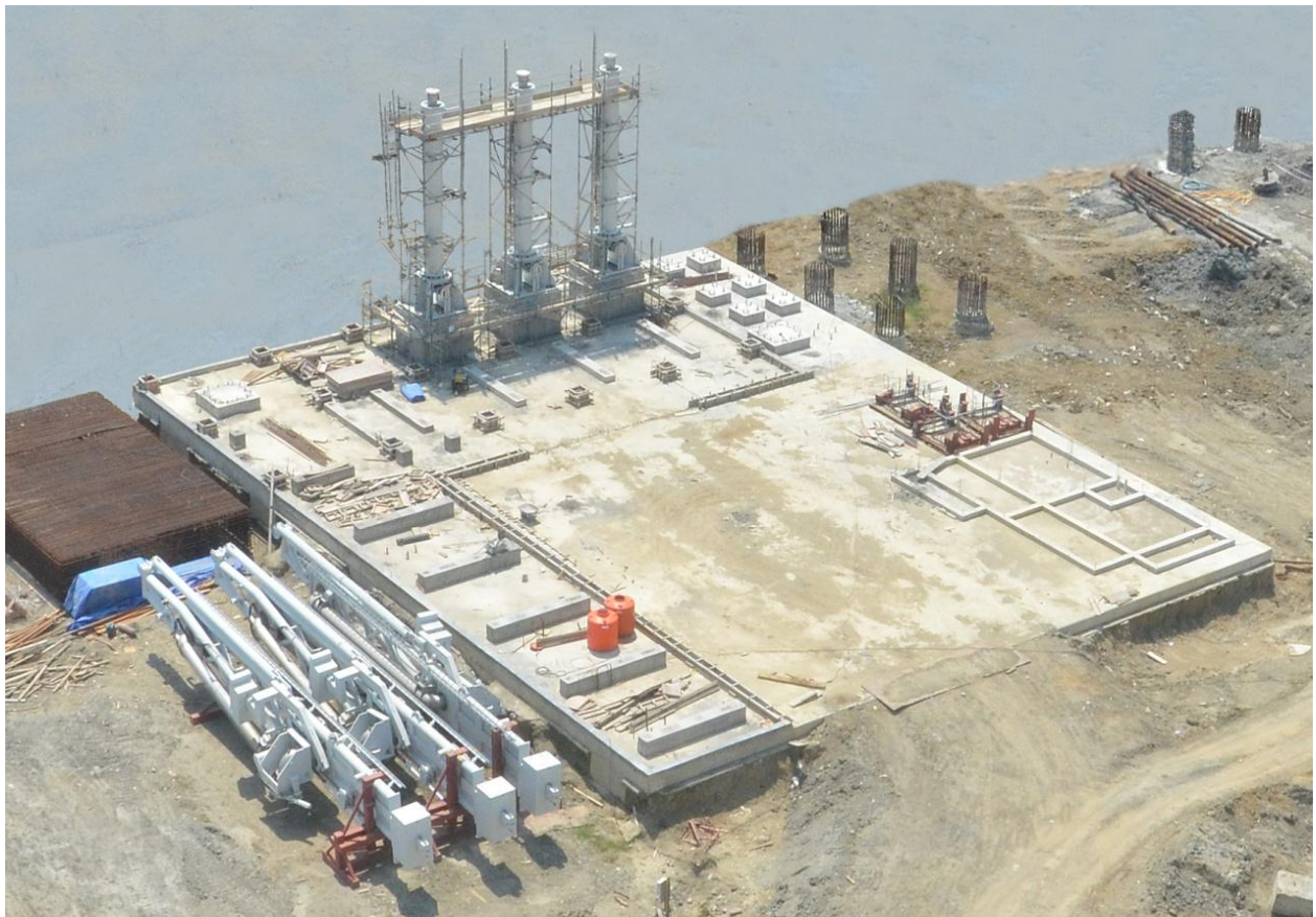
Jetty Loading Platform with erection of Hydraulic Marine Loading Facilities in progress
