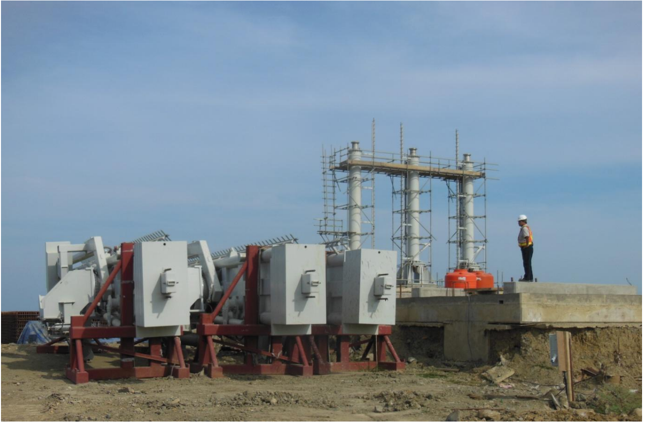
Jetty Loading Platform with erection of Hydraulic Marine Loading Facilities in progress
