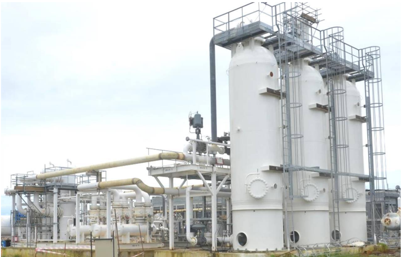
Erection & positioning of the Amine Contactor & the Mole Sieve Gas Dehydrators for Pre-treatment Train
