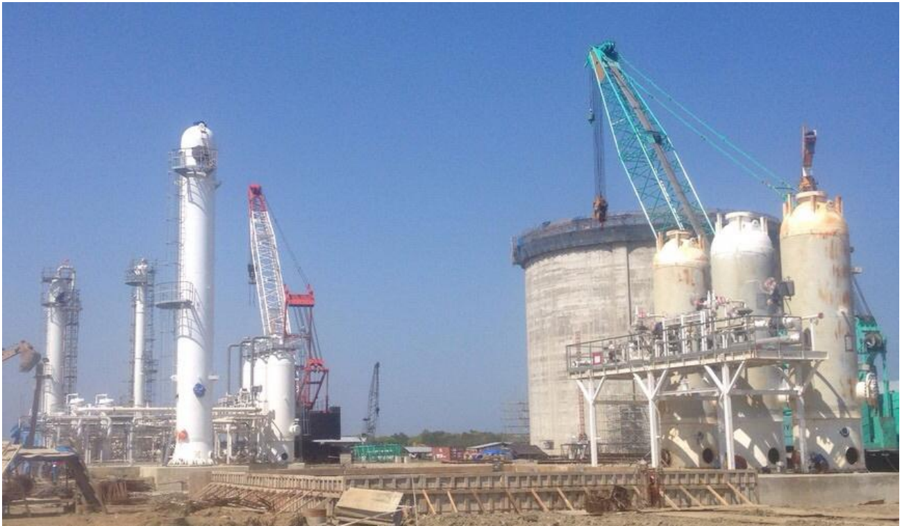
Erection & positioning of the Amine Contactor & the Mole Sieve Gas Dehydrators for Pre-treatment Train
