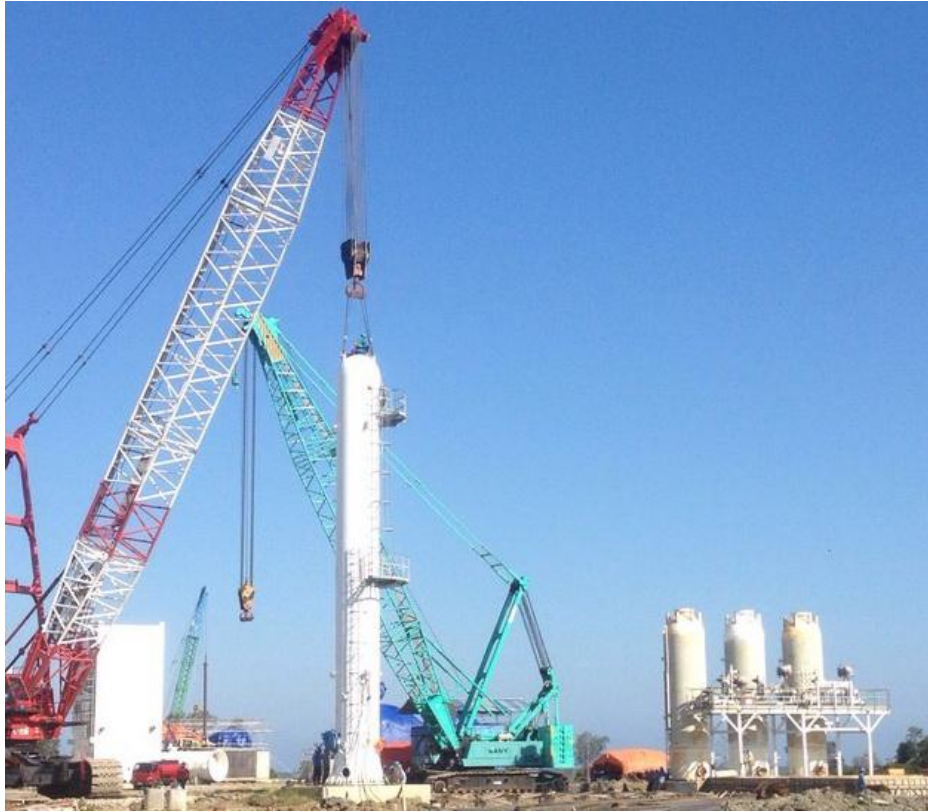
Erection & positioning of the Amine Contactor & the Mole Sieve Gas Dehydrators for Pre-treatment Train
