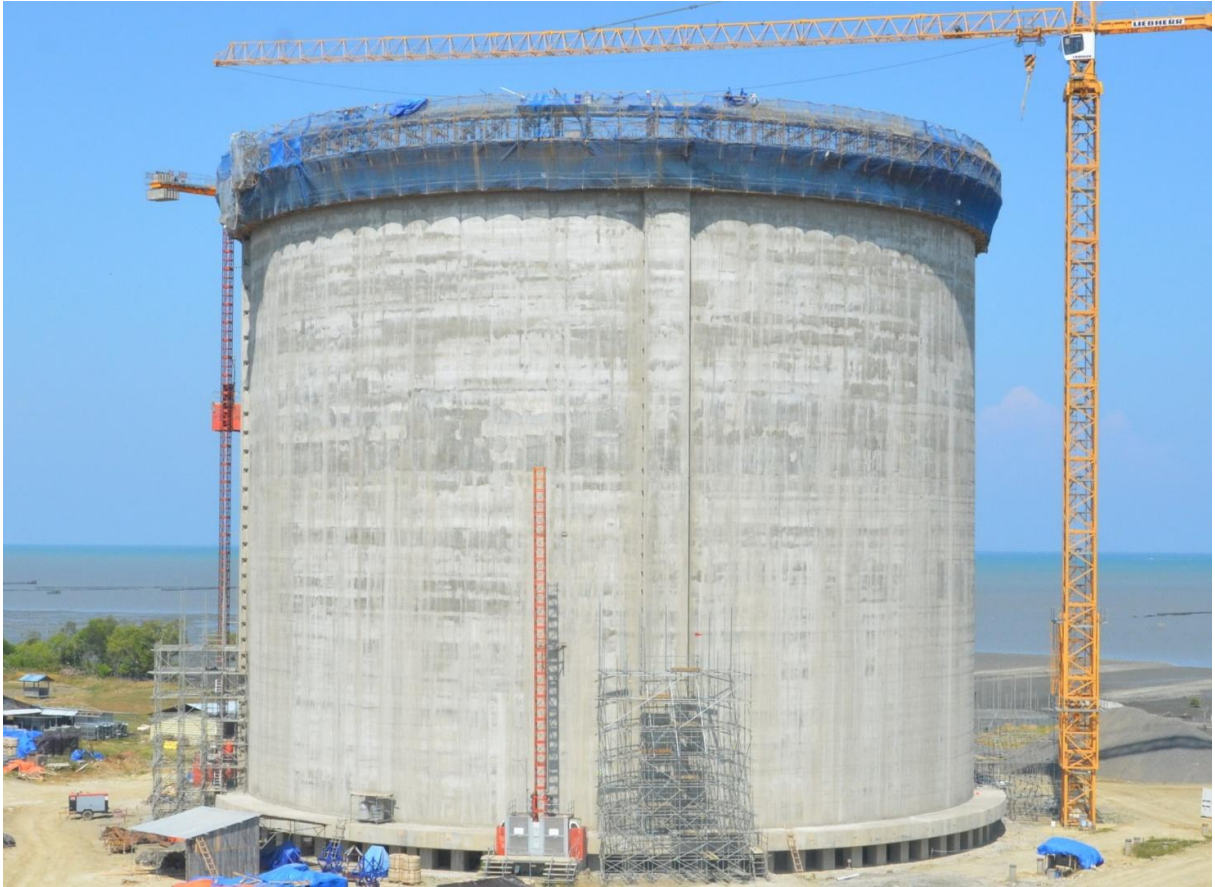
Slipform of Tank Wall and Ring Beam for the 88,800 m 3 LNG Storage Tank completed
