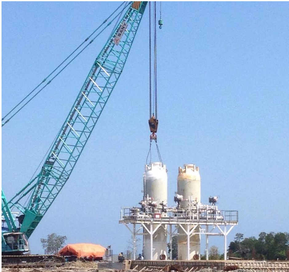
Erection & positioning of the Amine Contactor & the Mole Sieve Gas Dehydrators for Pre-treatment Train
