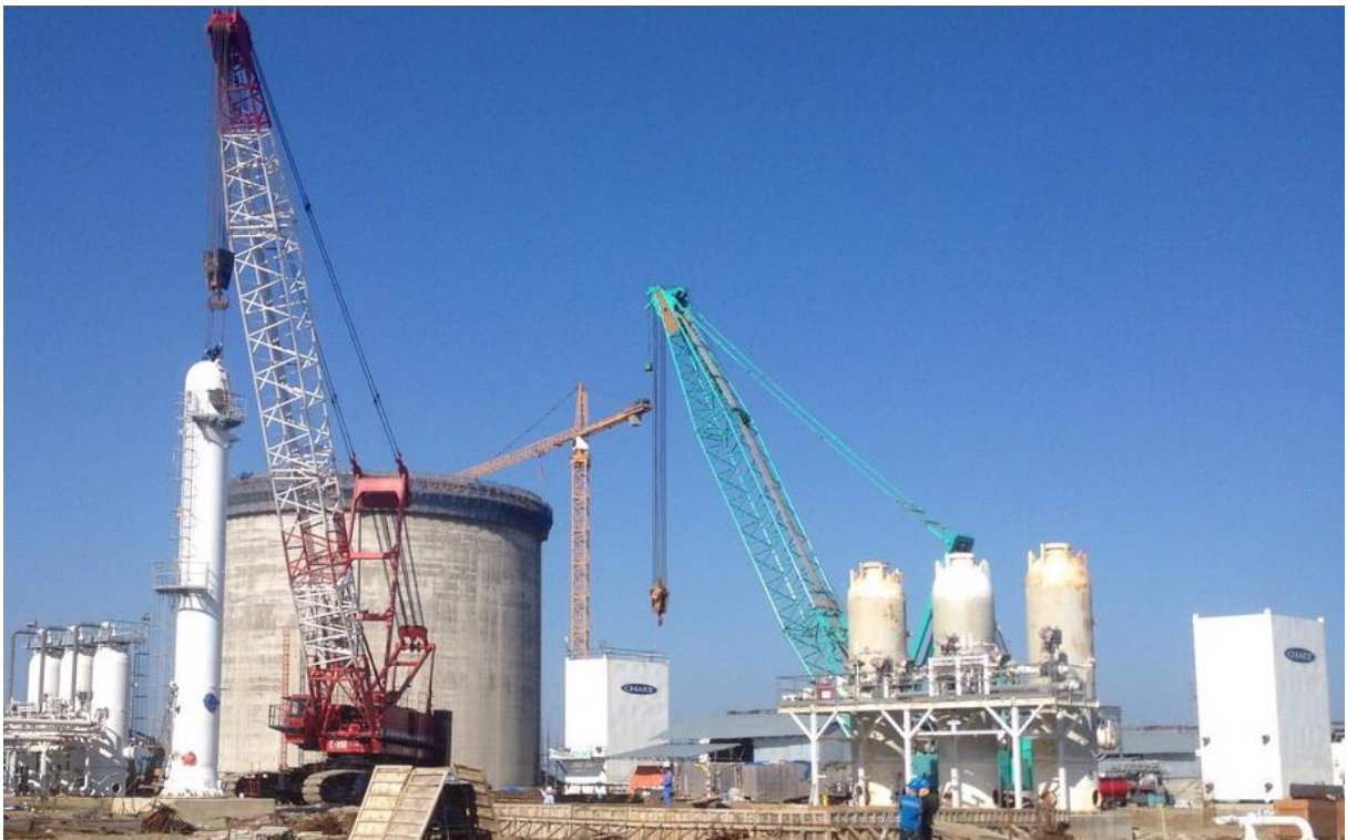
Slipform of Tank Wall and Ring Beam for the 88,800 m 3 LNG Storage Tank completed
