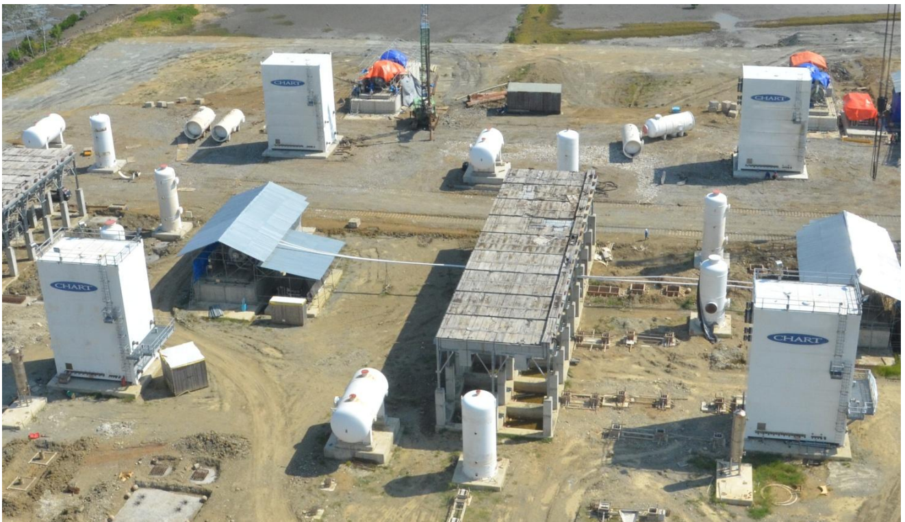
Overview of the 4 x 0.5MTPA Compression & Liquefaction Trains
