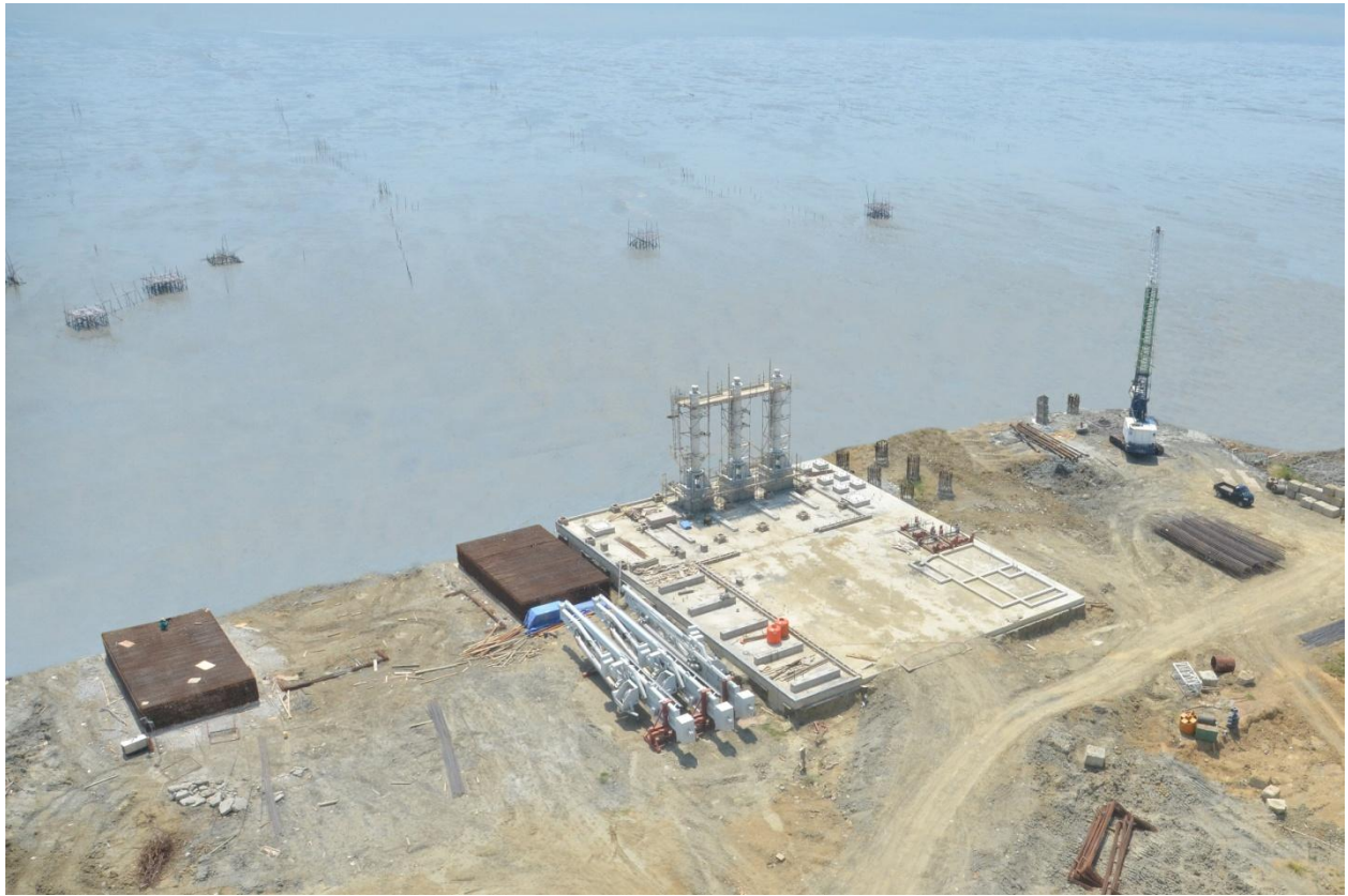
Jetty Loading Platform with erection of Hydraulic Marine Loading Facilities in progress
