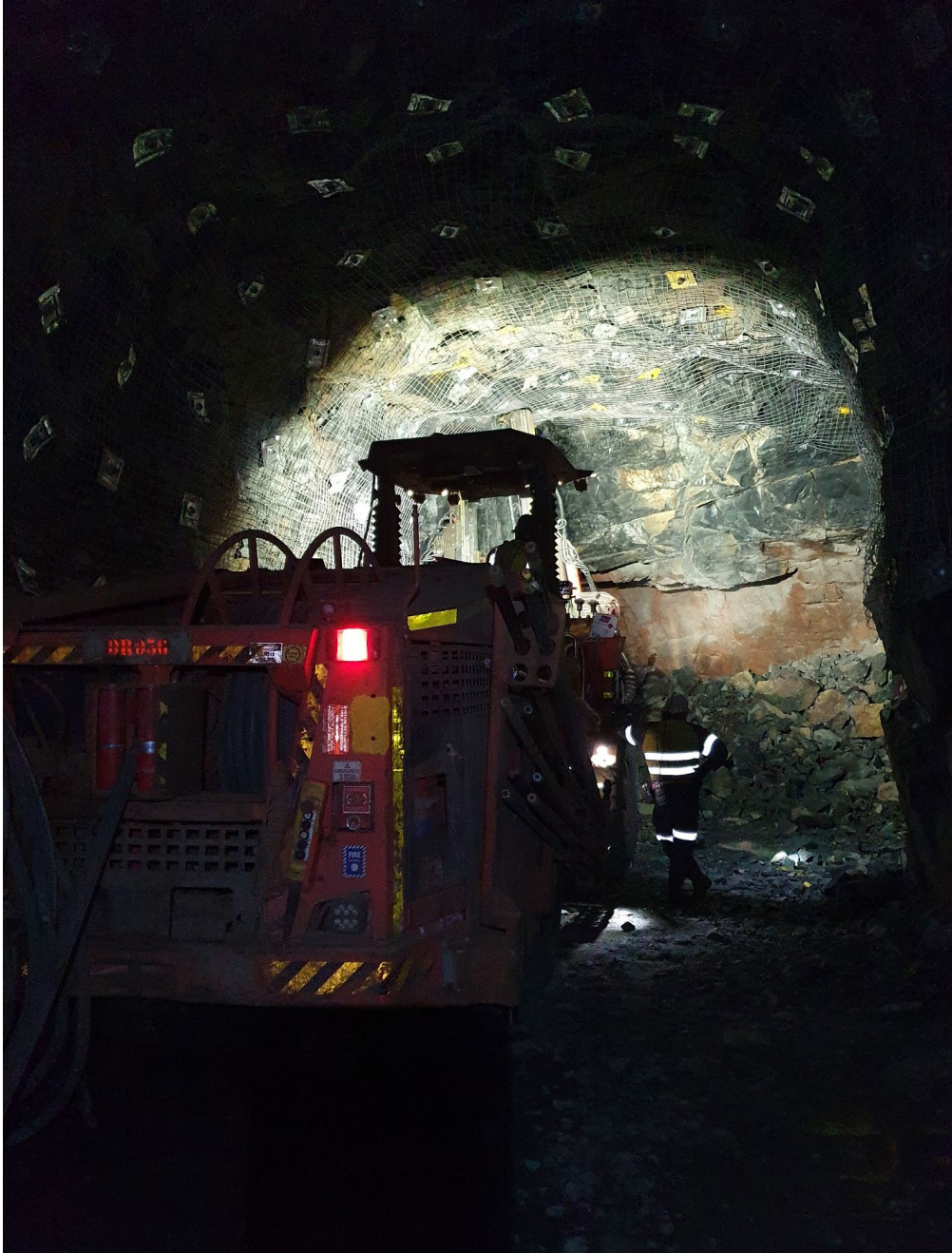
Figure 8: Development Jumbo at the breakthrough cut into the historical decline.
