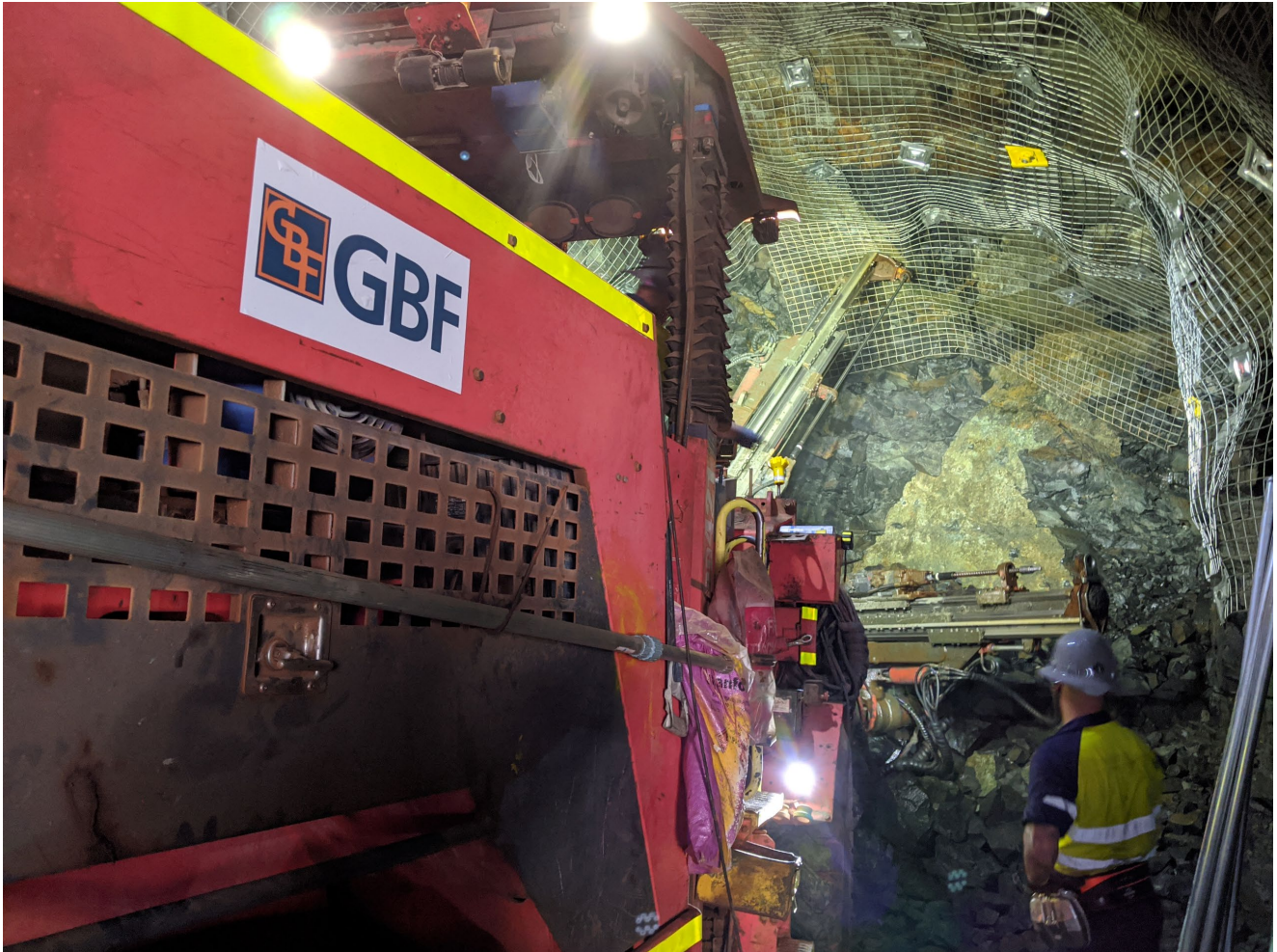
Figure 7: Development Jumbo installing ground support in the new Paris Decline.
