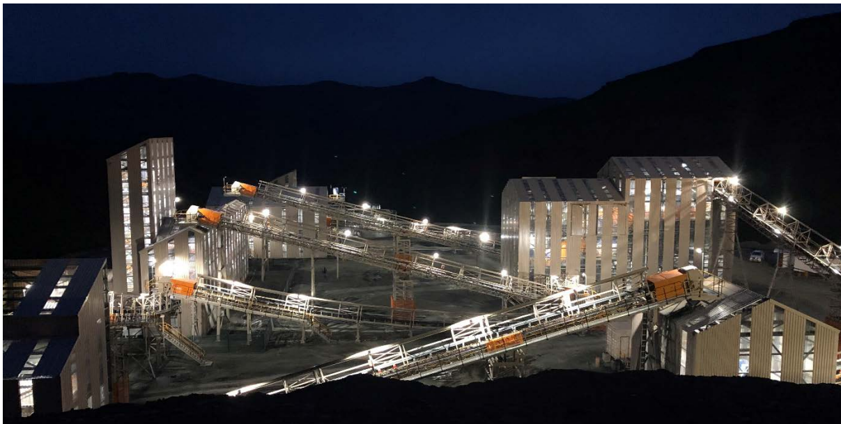
The Mothae 1.1 Mtpa commercial treatment plant
