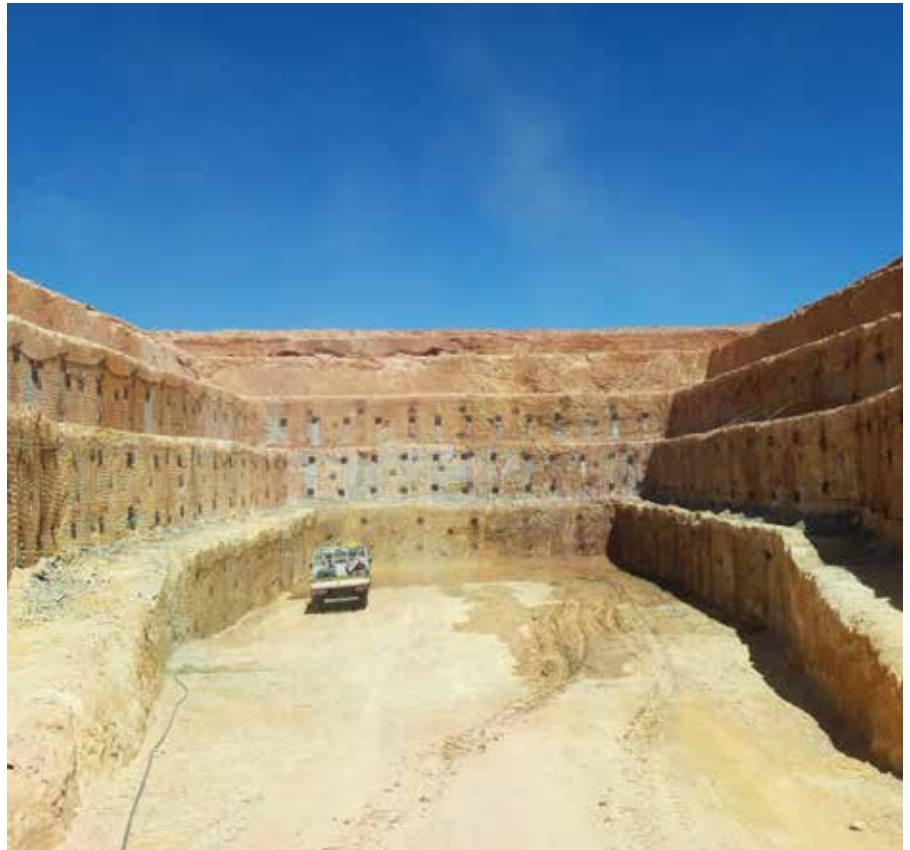
Completed box-cut for shaft collar civils.
