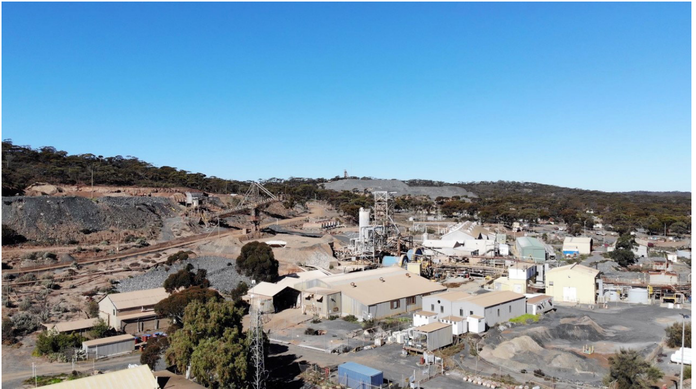
Existing Norseman Project administration and processing complex.
