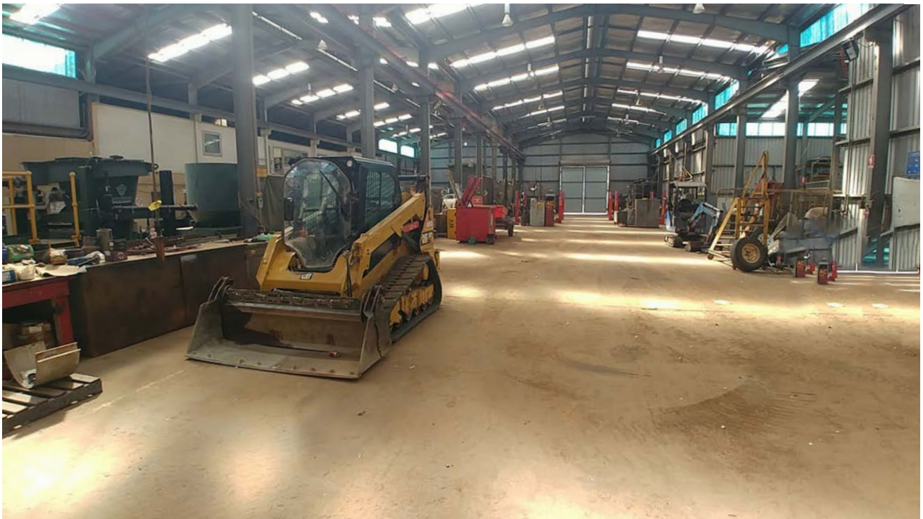
Existing workshop infrastructure.
