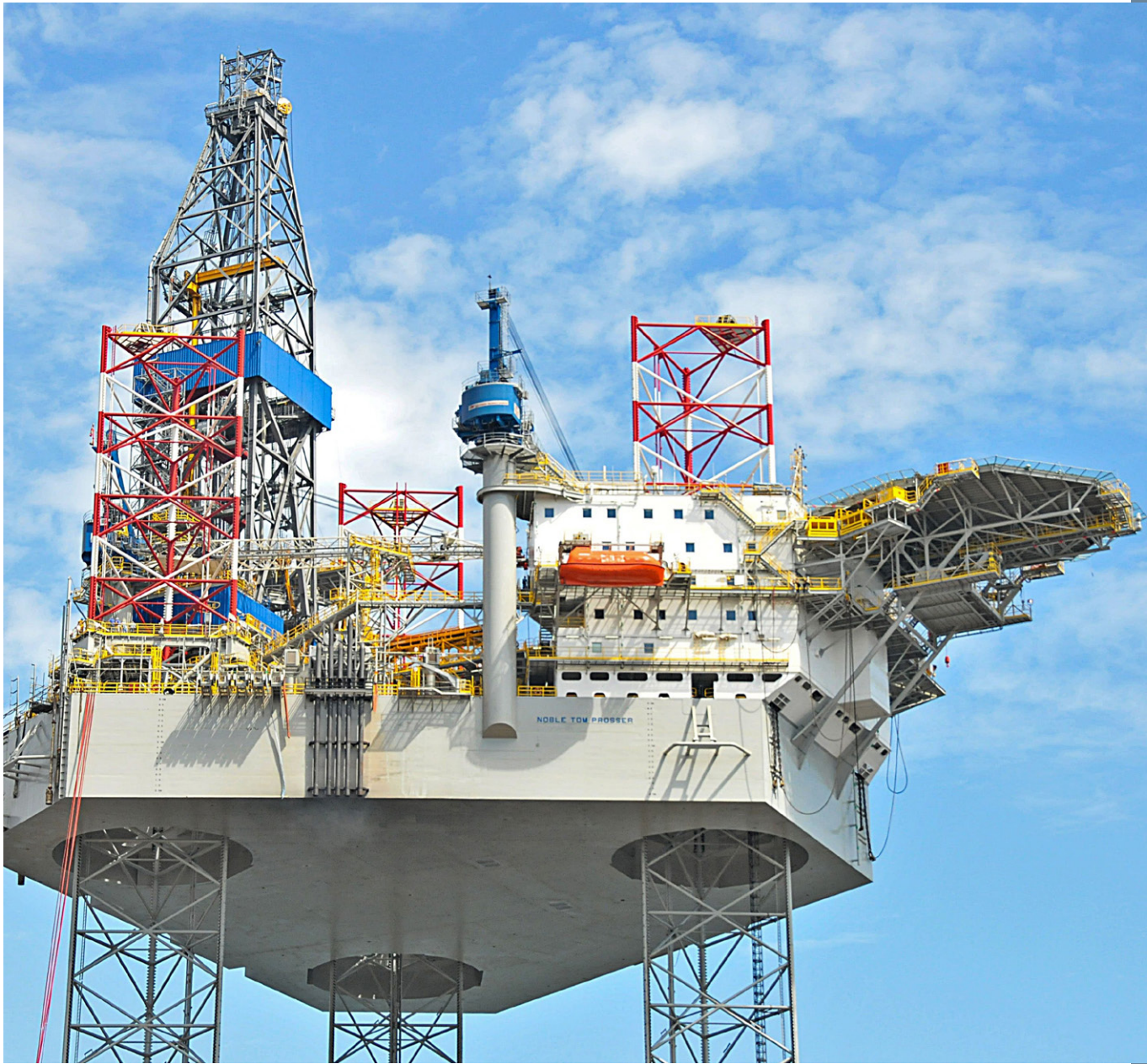
The Nobel Corporation's Tom Prosser rig utilised in the Dorado drilling campaign
