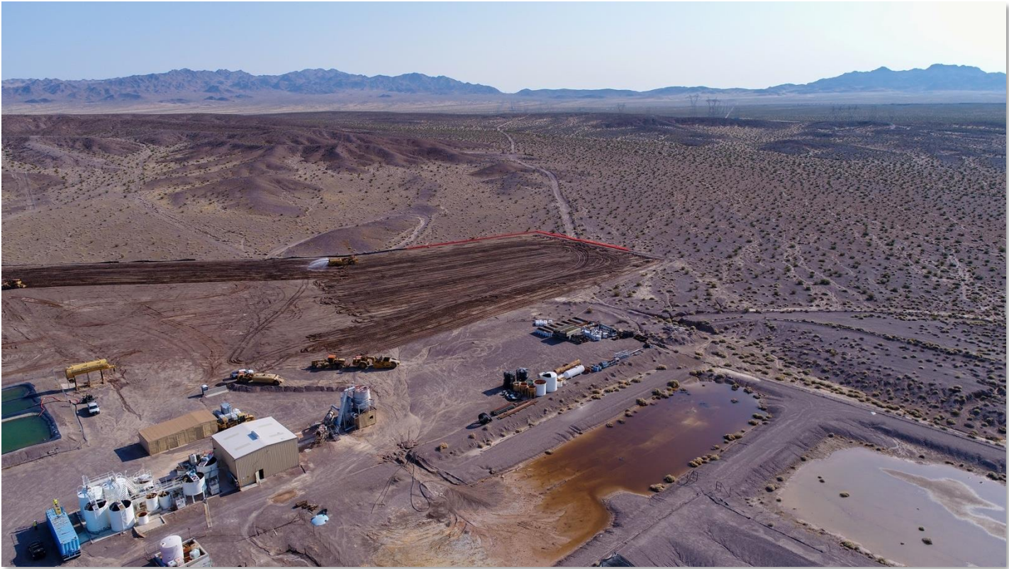
Figure 1: Aerial photo of early site works
