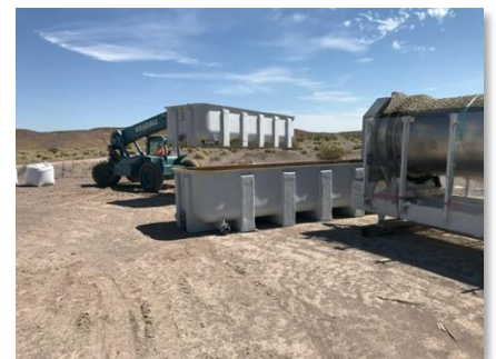
Figure 4: Photo of solvent extraction (SX) equipment being unloaded on site
