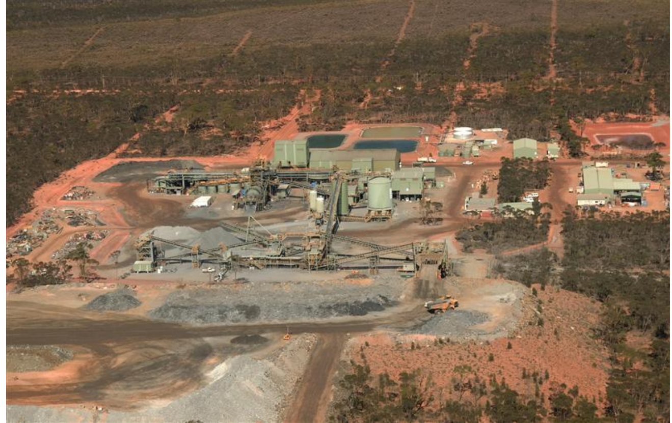
Lake Johnston process plant
