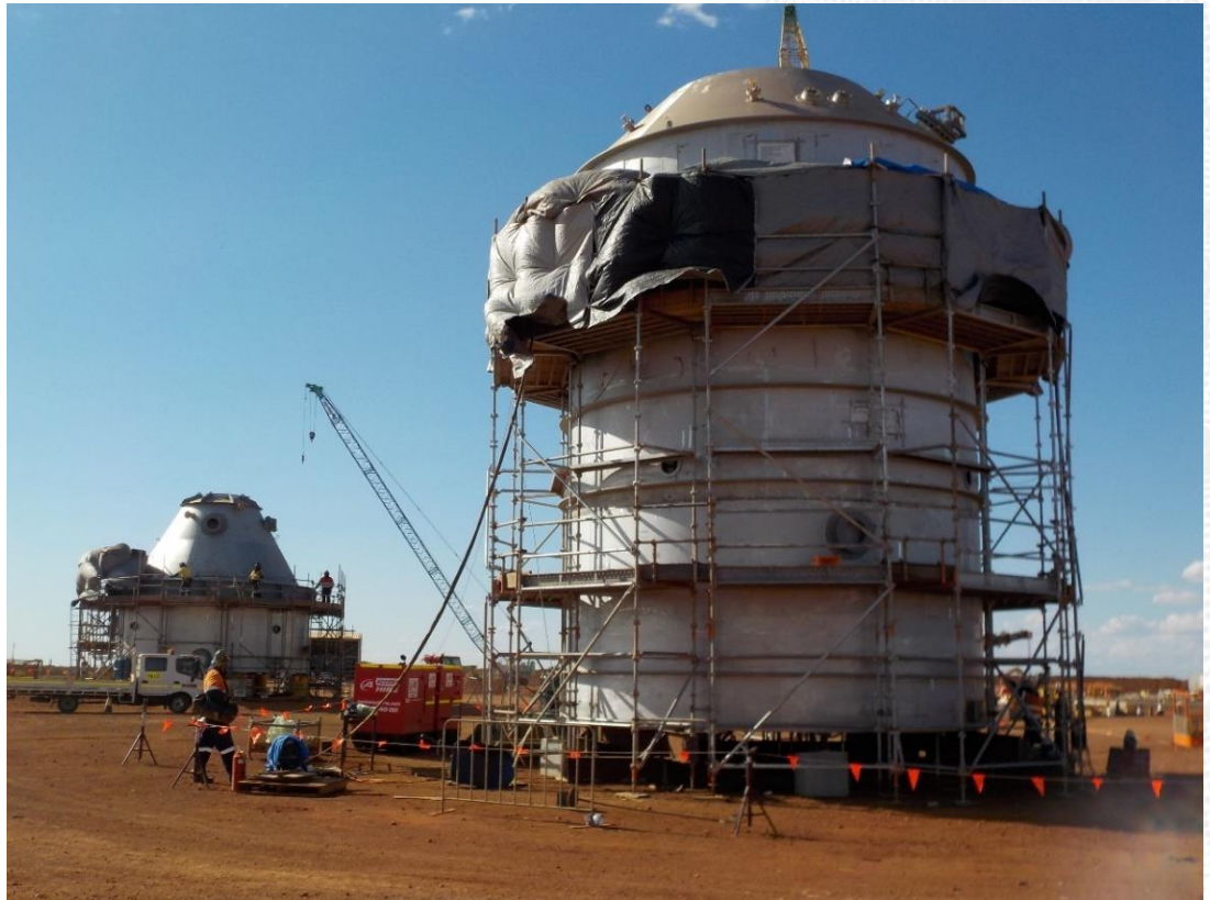
Figure 9: Tank fabrication
