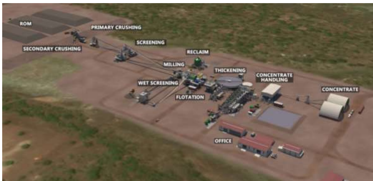
Figure 5: Rendered View of the Process Plant
