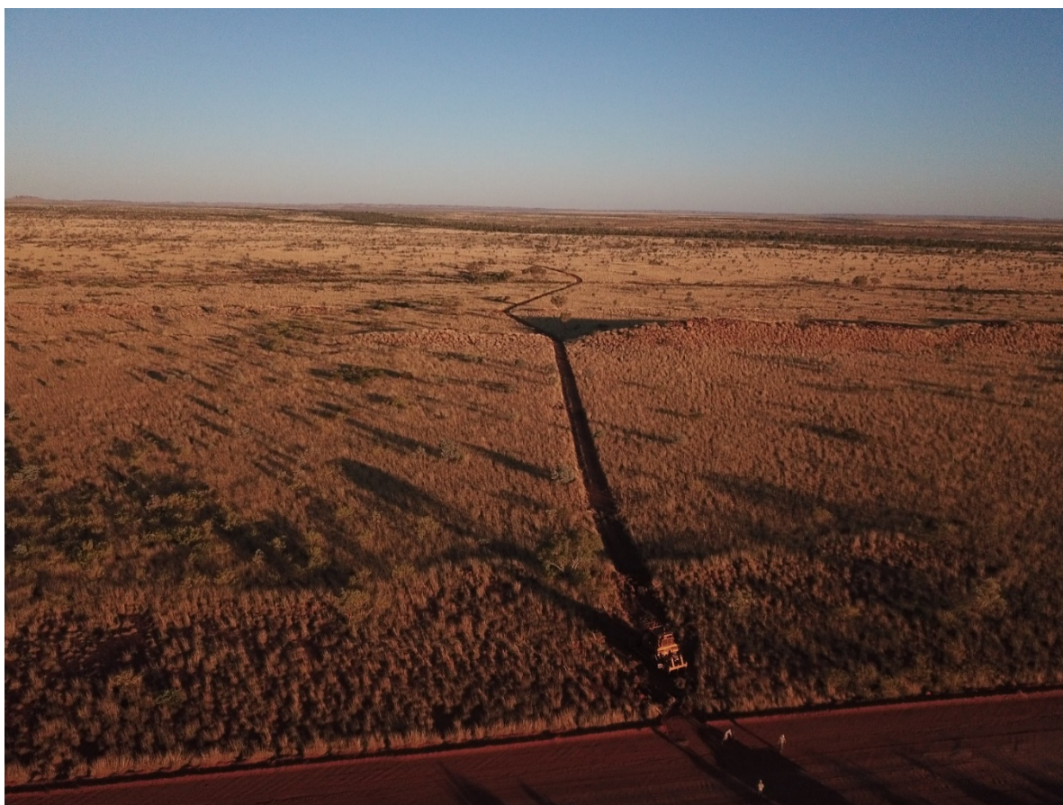
Figure 1: New access road construction commenced
