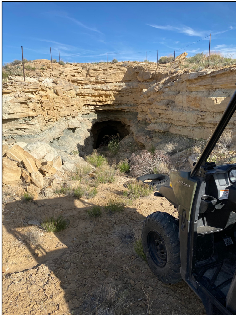
Figure 4. Portal for largest historical mine within Section 36 with well over 300m of workings. Reported samples MLE20003 through MLE20007 came from mineralized material within this mine.
