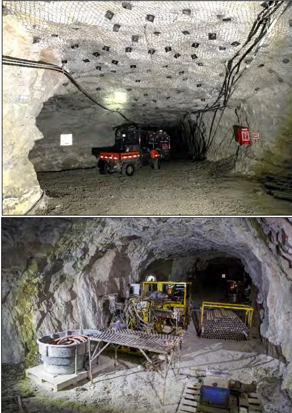
Photos 1 – 3 – Infrastructure at Oracle Ridge
