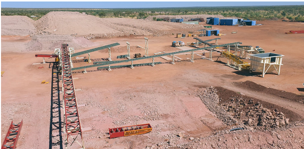
Ore Sorter system installation works have commenced at Browns Range.
