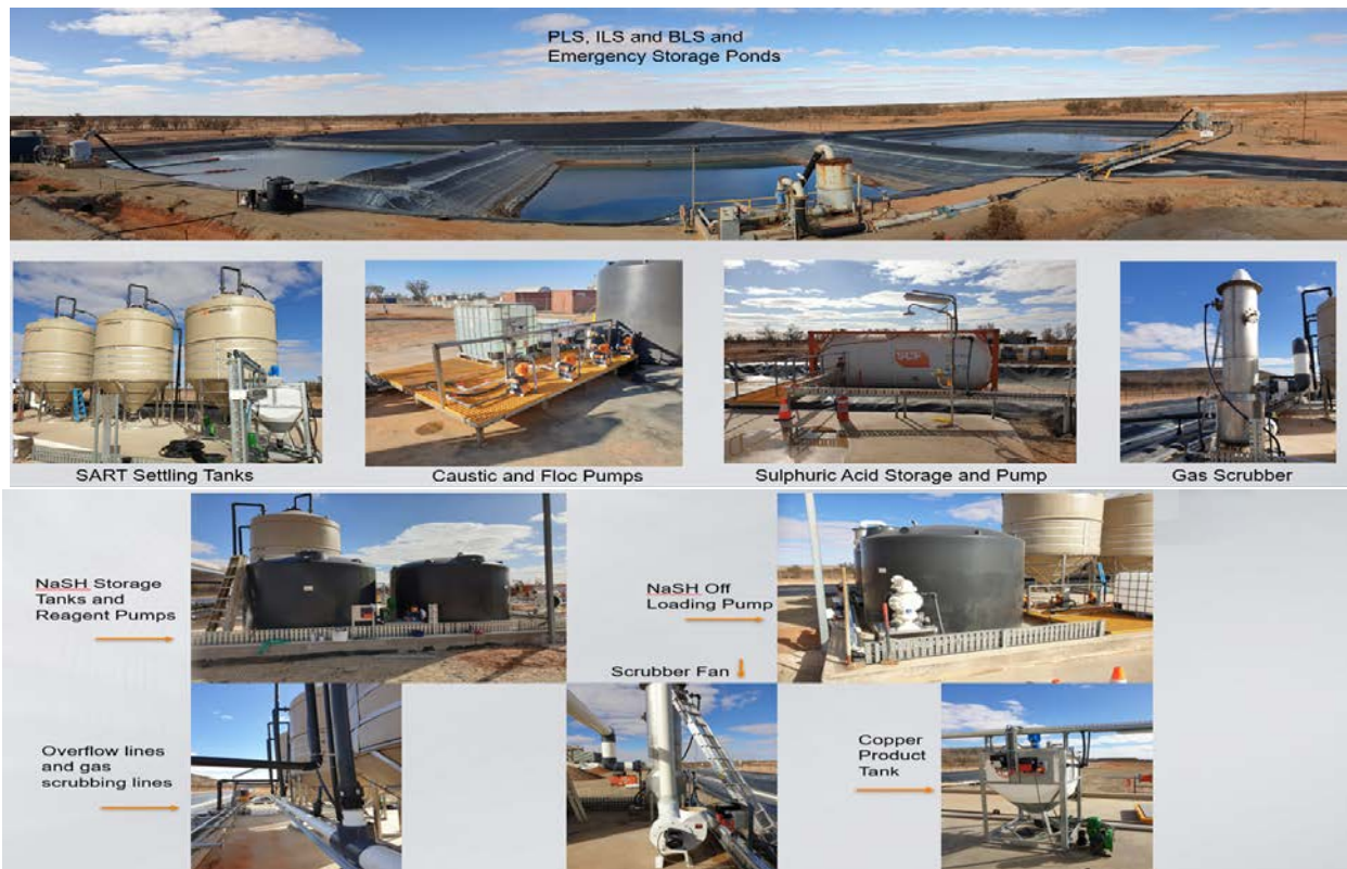
Photograph 2: Process ponds and new SART plant
