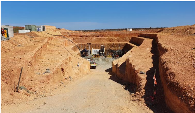
Raise bore machine set-up in box-cut
