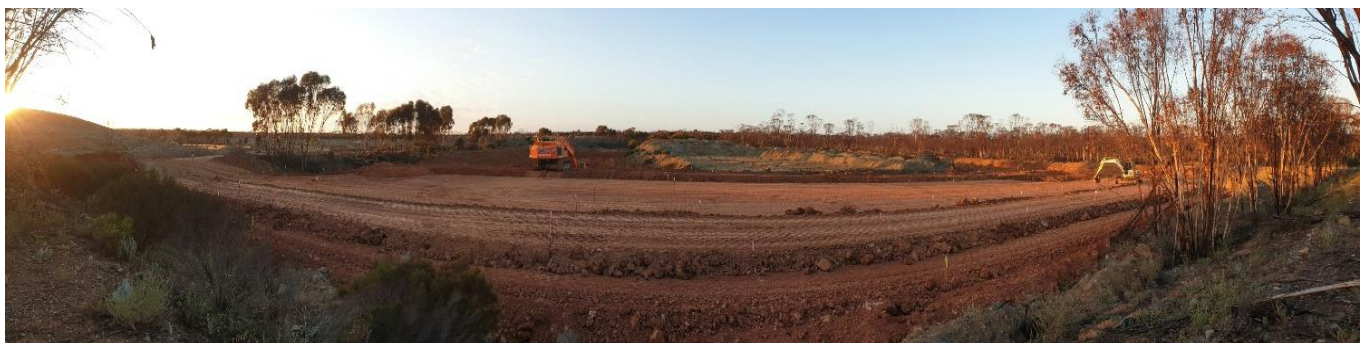
Heap leach pad construction
