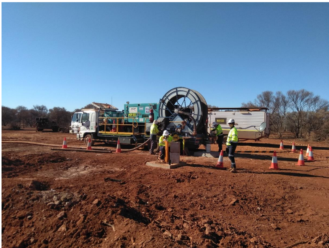
Figure 5: Water Production Bore Pump Testing
