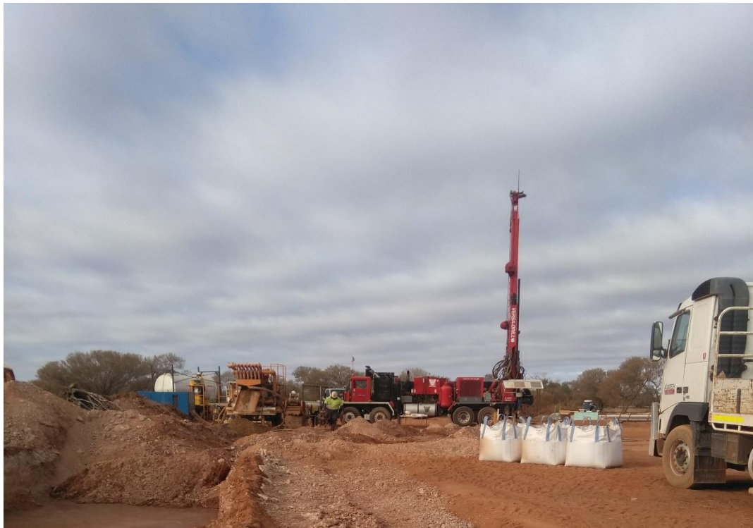
Figure 4: Water Production Bore Drilling
