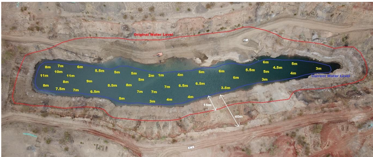
Figure 4: Pit dewatering continues.
