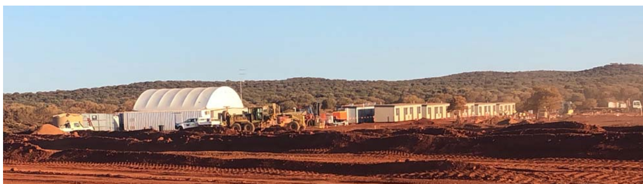
Figure 4: Construction of the KOTH village is underway.
