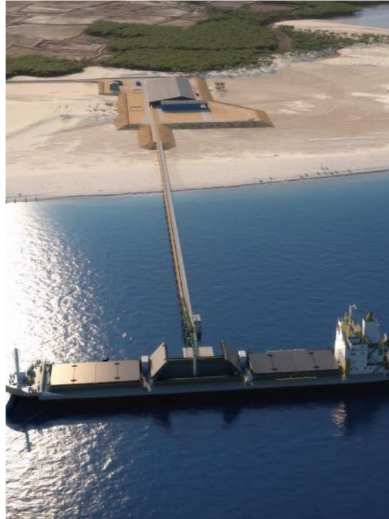
Critical path contracts
