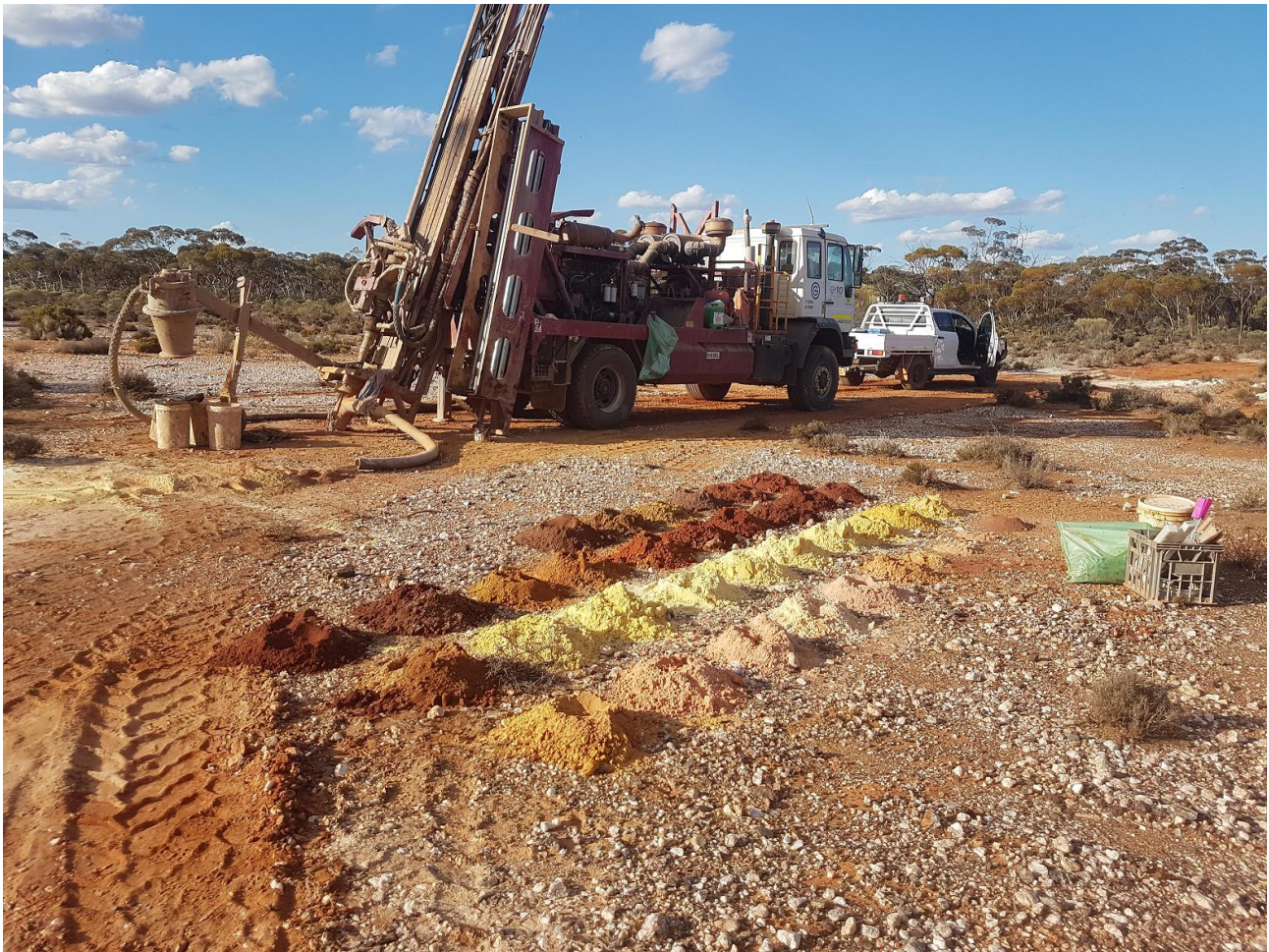
Figure 5: Air core drilling at North Kanowna Star
