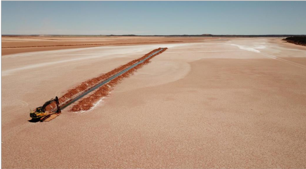
Figure 3.2: Trench Excavation (T Swierczuk, Feb 2020)
