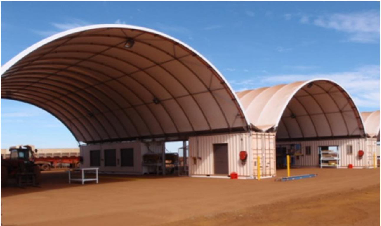
Figure 9.1. Typical Maintenance Workshop Area
