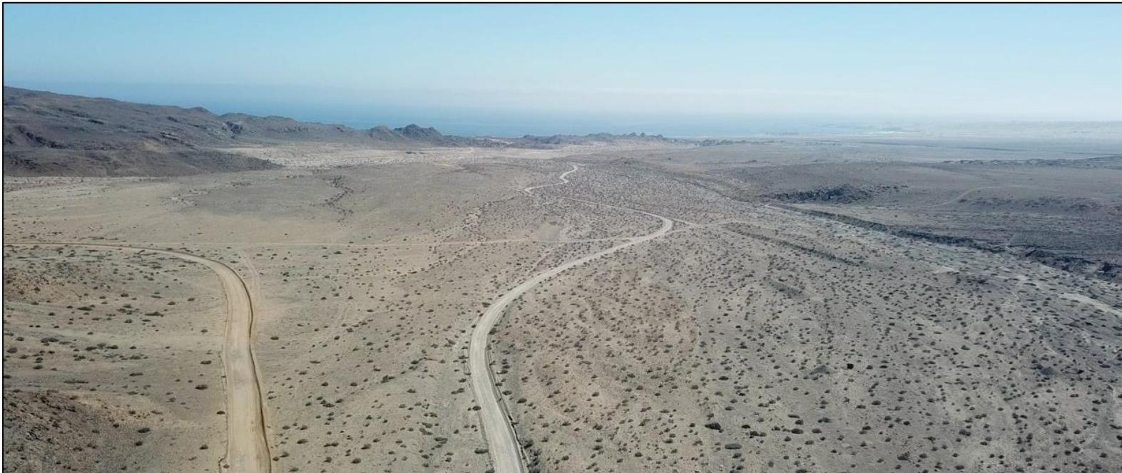
El Zorro access road looking west to Pacific Ocean & Pan American Hwy
