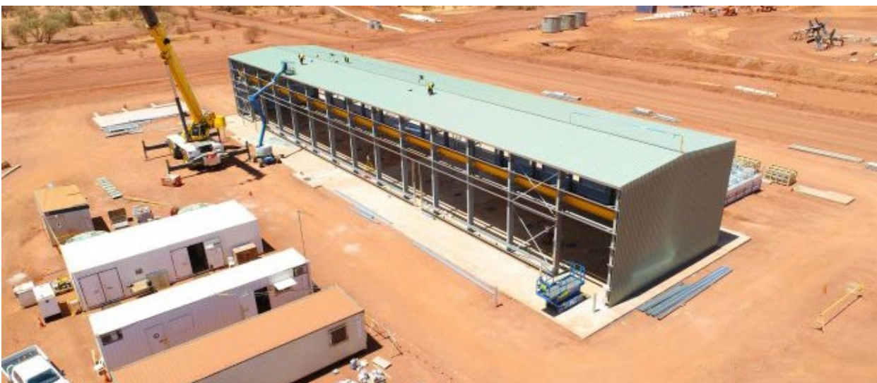
Power station construction
