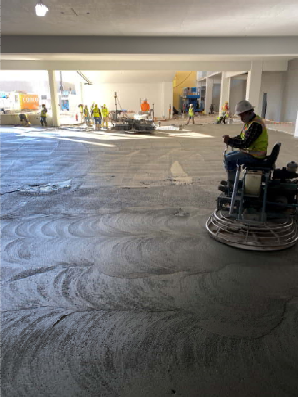
Figure 7. Slab on Grade being placed and finished
