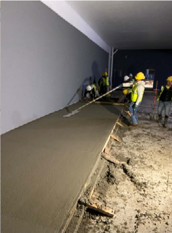
Figure 6. Interior sidewalk being finished
