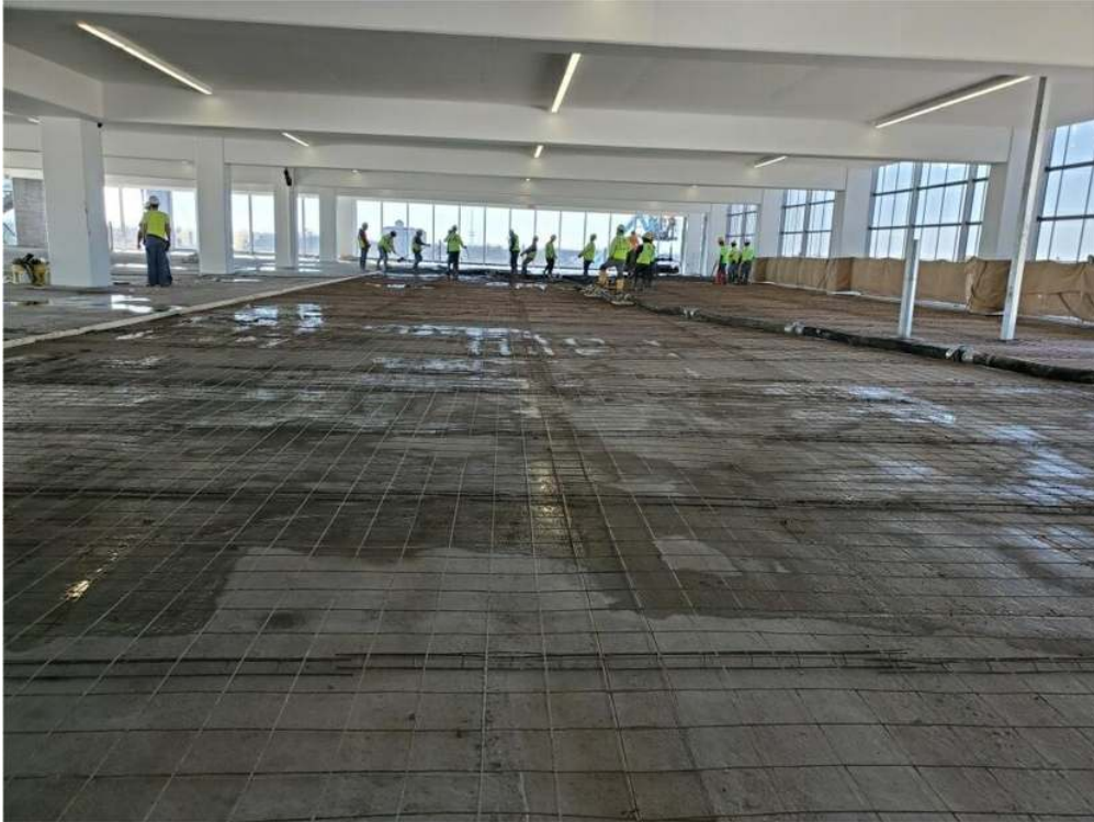
Figure 3. Laying EdenCrete® concrete overlay
