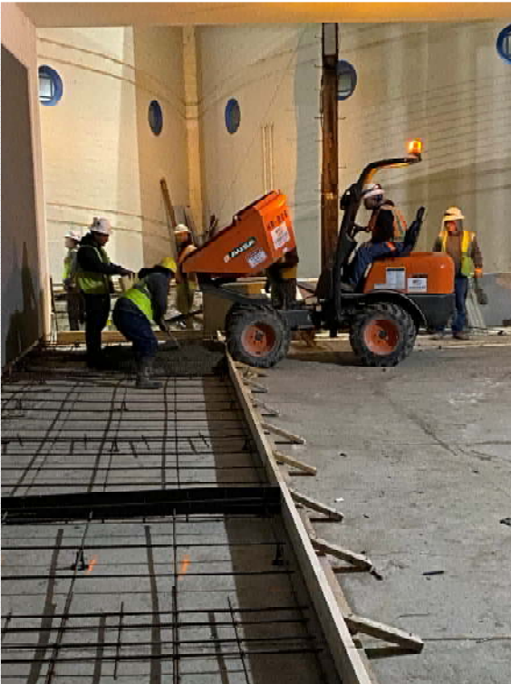
Figure 5. Interior sidewalk being installed
