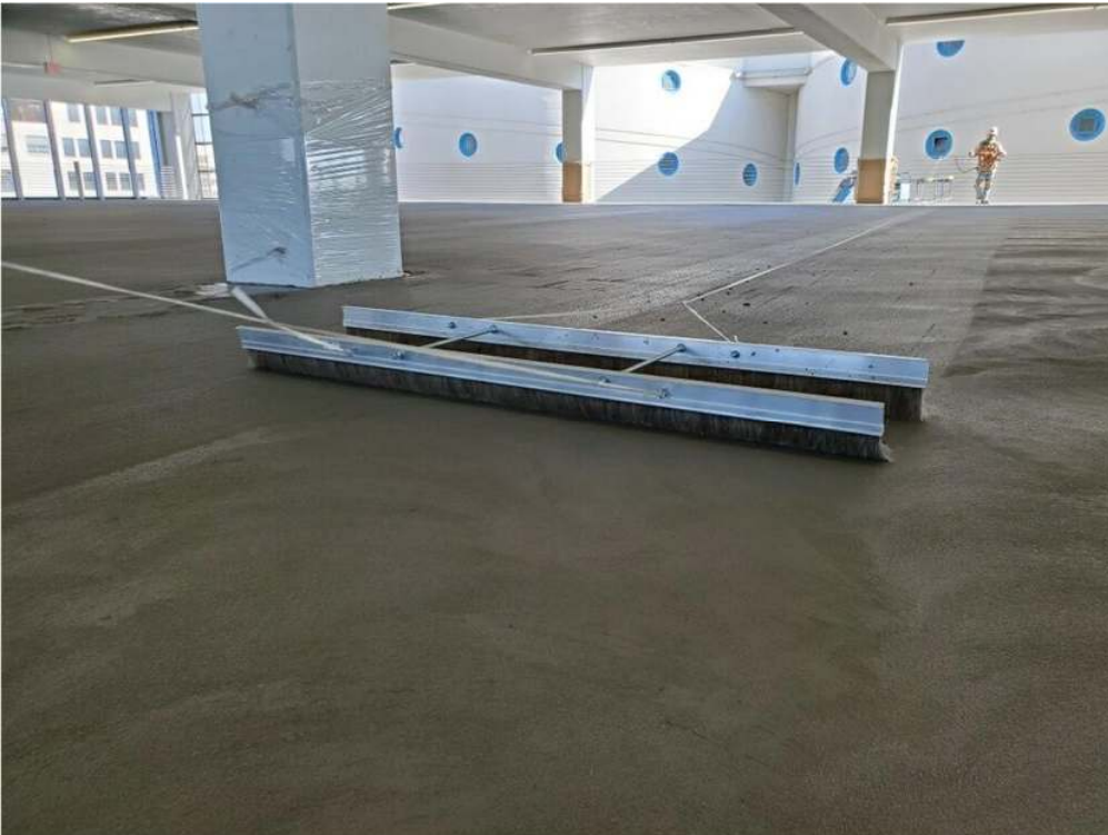
Figure 4. Applying suspended broom finish to the EdenCrete® concrete
