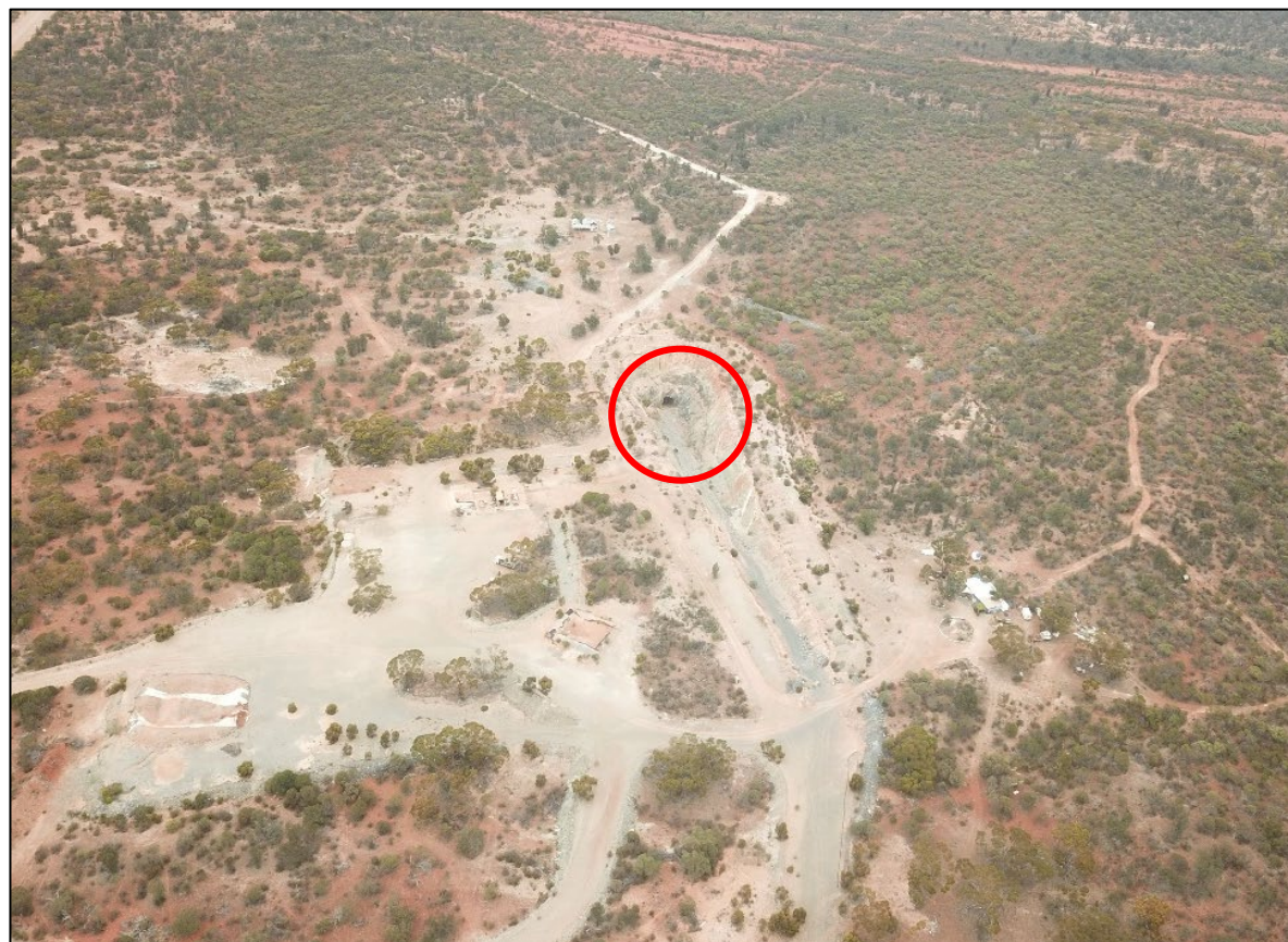
Figure 7: Aerial view of boxcut (circled) for entry to underground and the historical mining infrastructure across the First Hit Mining Project location
