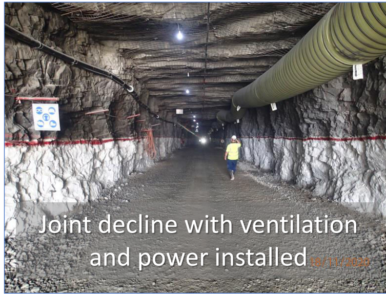
Joint decline splits after 152m to Lando (left) and Kundu (right) declines of 4m x 4m. Hanging and side walls are competent granite and very stable
