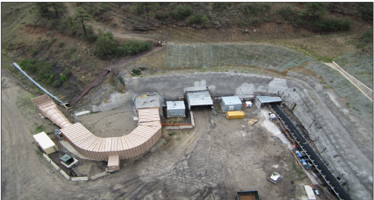
Image: Blue seam portal entries left to right: fan; personnel and materials; and belt.
