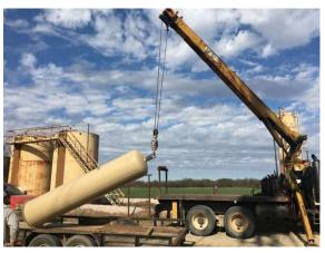
Figure 1. Delivery and installation of a new separator on location, Thelma Well, SCOOP Play, Oklahoma
