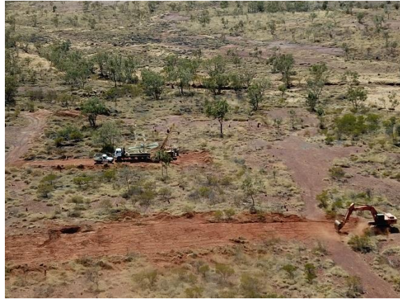
Photo 4. Drill pad construction at the Trump
