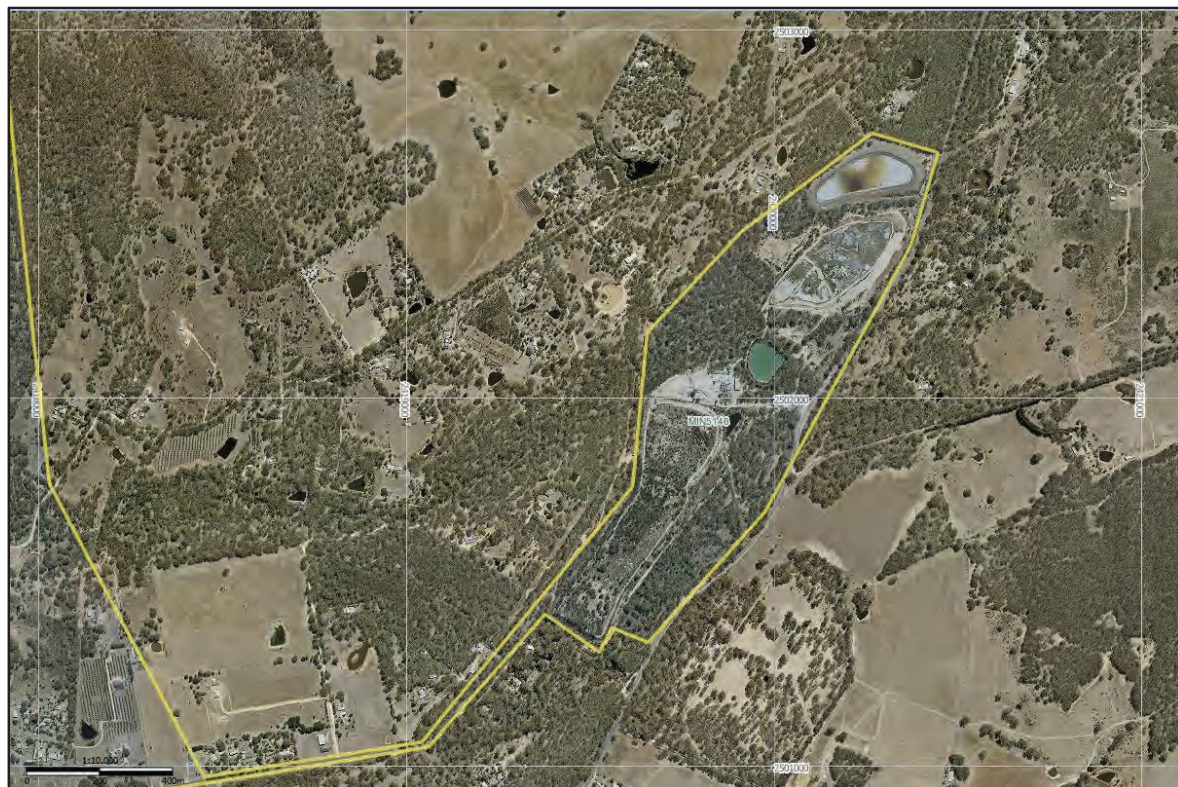
Figure 3-2 Aerial Photograph of Porcupine Flat Process Plant (GSV taken 02 2017)
