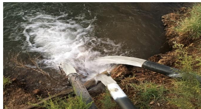
Photo 8. Transfer pump and bore pump discharge.
