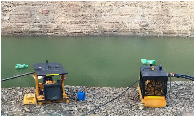
Photo 5. Pit dewatering pumps in action.
