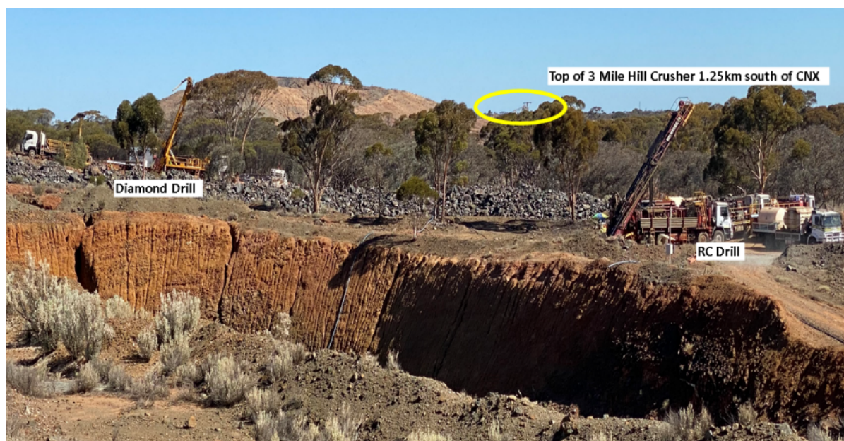
Figure 8: View South toward 3 Mile Hill Crusher/ROM with drilling underway at CNX (14/12/2020)
