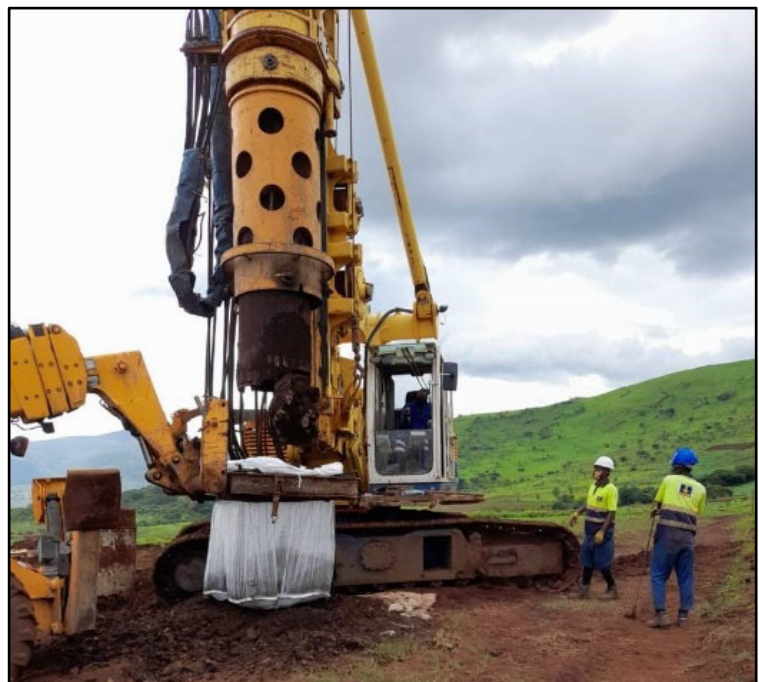
Figure 4: large diameter drill rig in operation, December 2020
