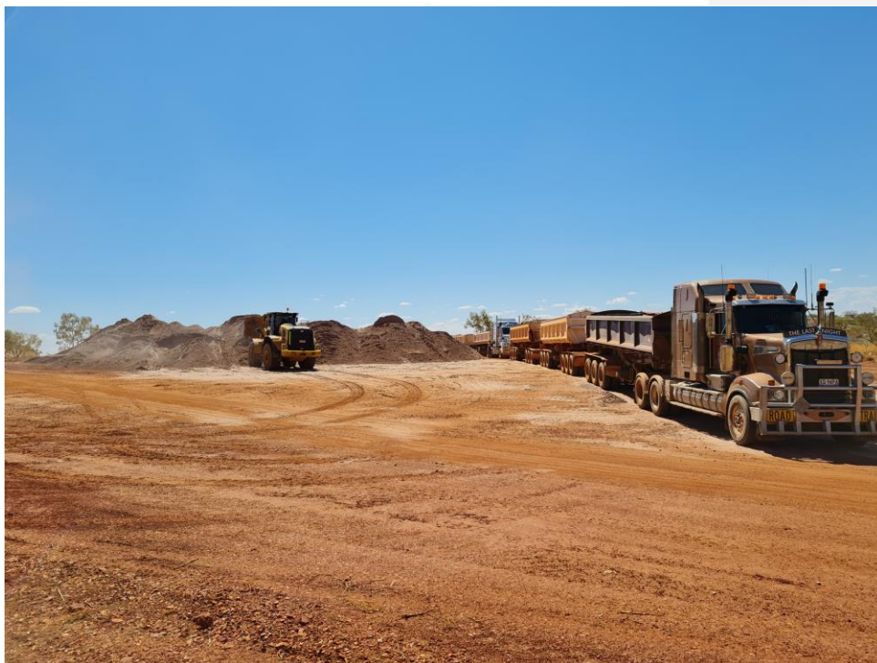
Figure 2 Tick Hill Tailings Dam Stockpiles being loaded and hauled to 3 rd party processing facility.
