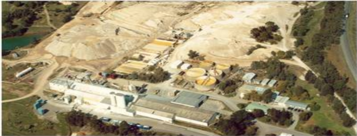
Figure 2: Aerial of Pittong processing plant facilities
