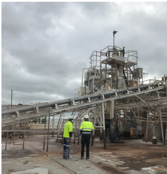
Figure 3: Pittong processing plant facilities
