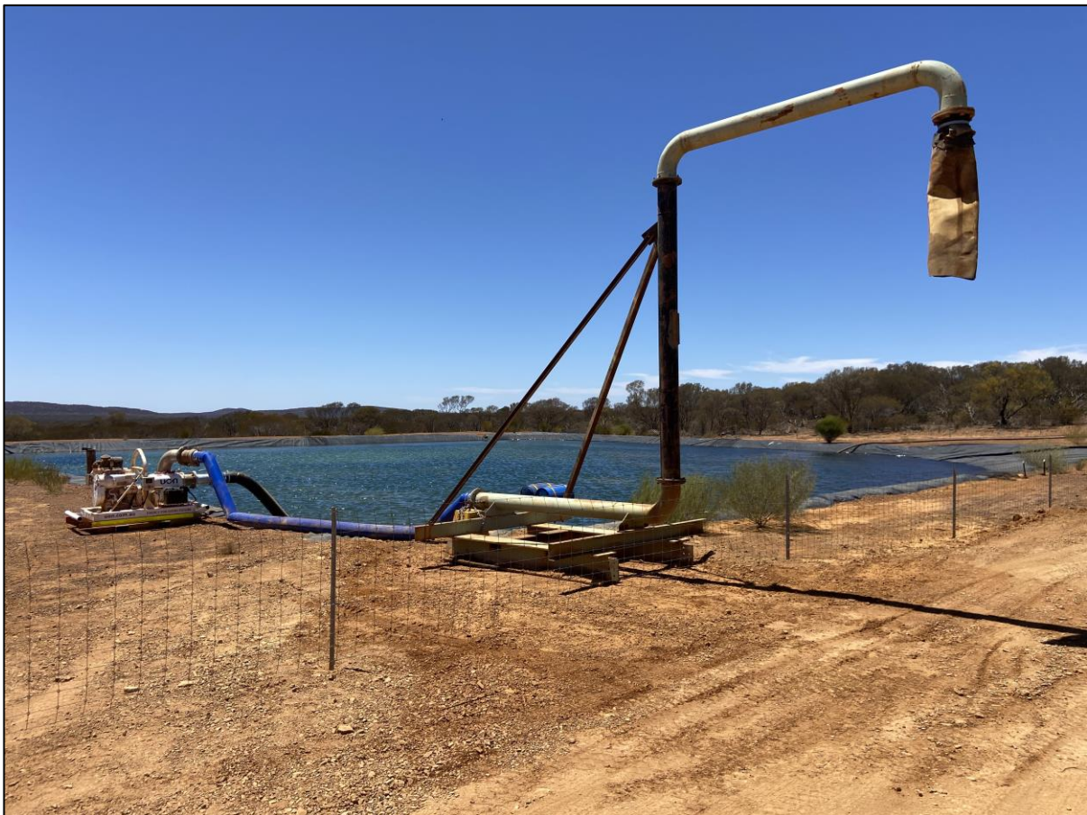
Figure 2: Site water supply established at the Shine Iron Ore Project as part of early siteworks.
