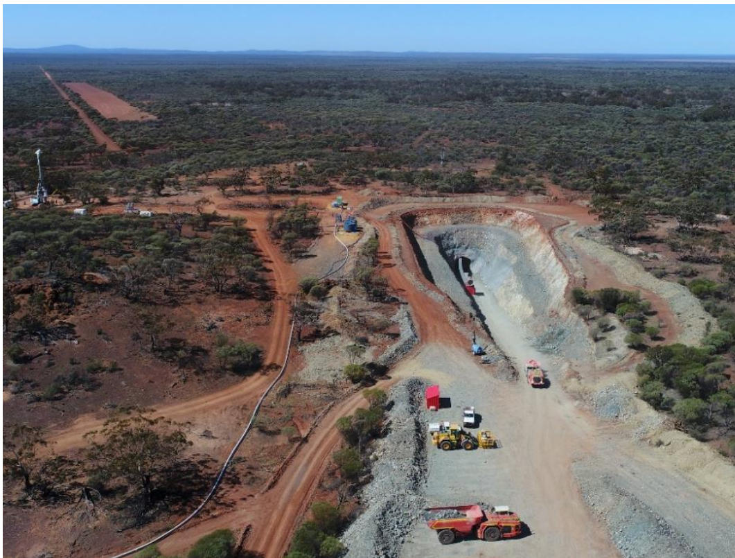
Figure 5: Rothsay boxcut with airstrip in the background
