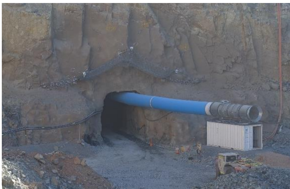
Figure 3: Deflector South West portal
