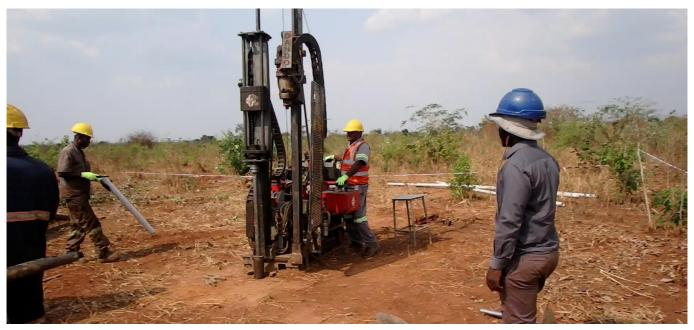
Figure 3. Push-tube core drilling at Kasiya.
