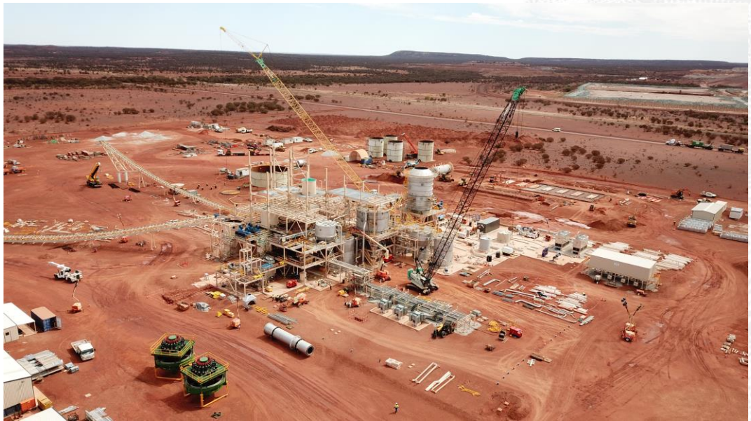
Figure 6: Aerial view of process plant site
