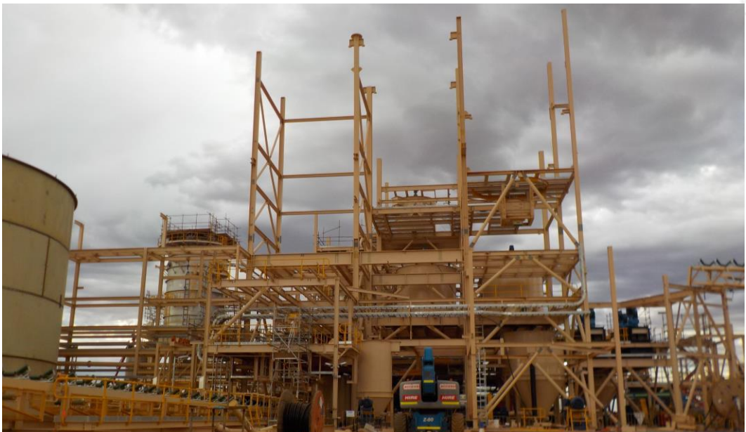
Figure 7: Process Plant structural steel erected to the 6th floor
