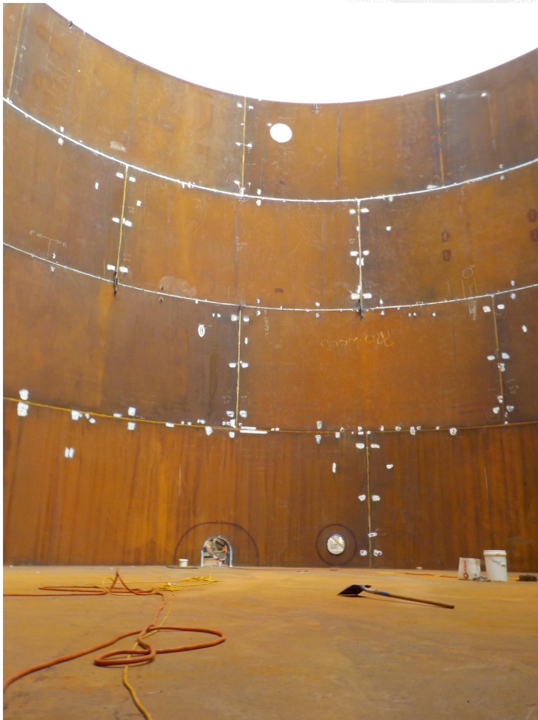
Figure 8: Flotation tank welding well advanced
