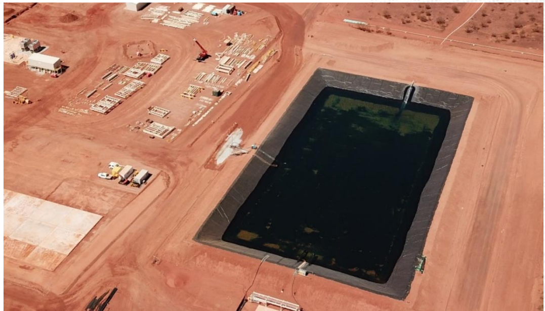
Figure 9: Raw water pond filling and commissioning has been completed
