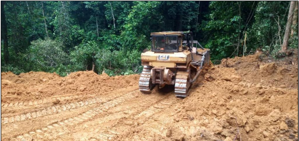
Figure 8 – Current Drill Pad Clearing
